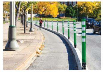
Pre-cast or cast-in-place concrete curb
