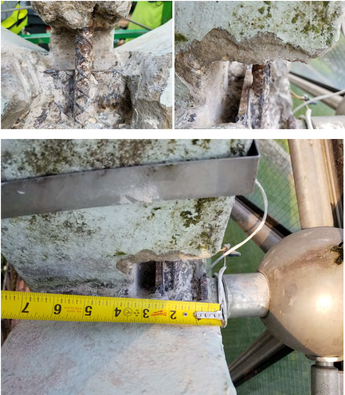
Figure 25: Opening of Weld Plate F in Area M.
