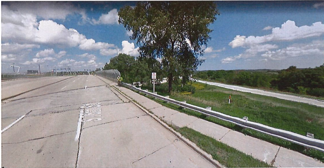
<Image Capture of Existing Condition at northbound bridge Looking North-Sept 2018 @ 2019 Google>
