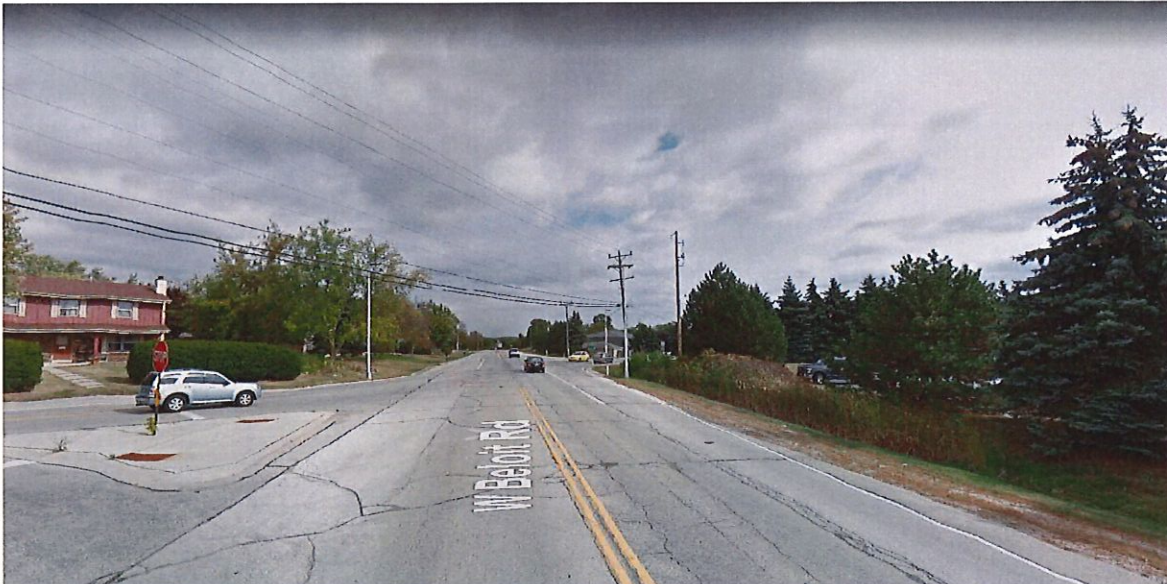
<Image Capture of Existing Condition at Coldspring Rd Looking East-Oct 2017 @ 2019 Google>
