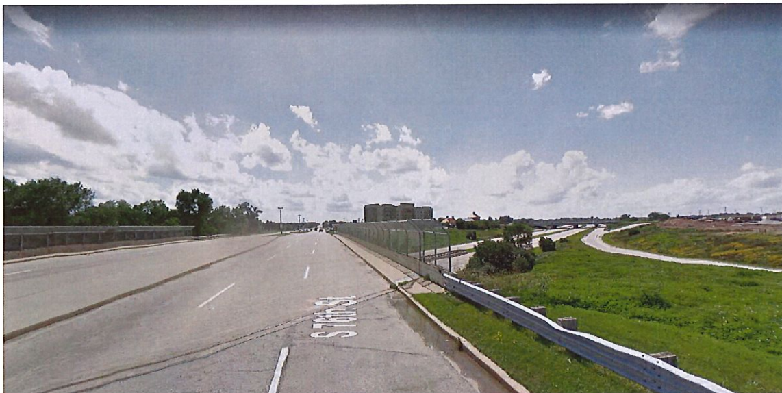
<Image Capture of Existing Condition at southbound bridge Looking South-Sept 2018 @ 2019 Google>
