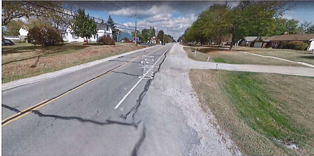
<Image Capture of Existing Condition at S. Willow Dr. Looking North-Sept 2017 @ 2019 Google>
