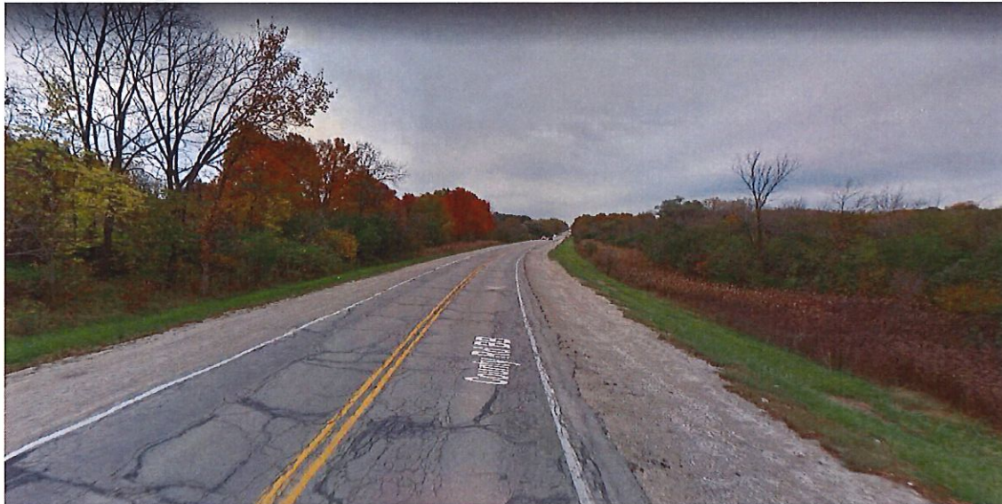
<Image Capture of Existing Condition at 9901 Looking East-Oct 2016 @ 2019 Google>
