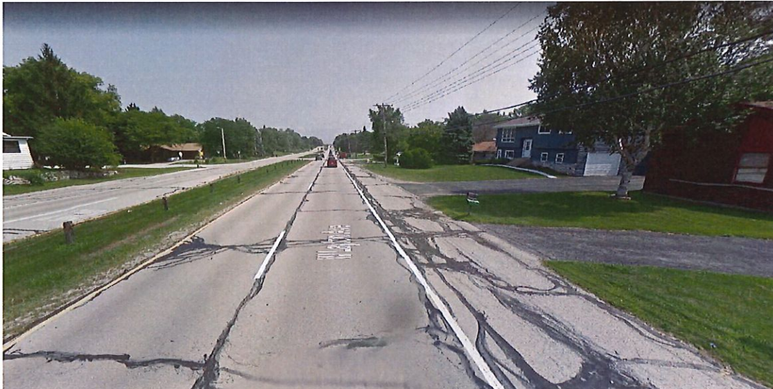
<Image Capture of Existing Condition at 3800 Looking East-Oct 2017 @ 2019 Google>
