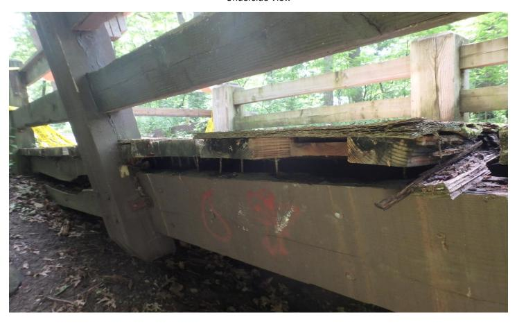
Rotted and Failed Railing, Wood Deck, and Fascia Beam
