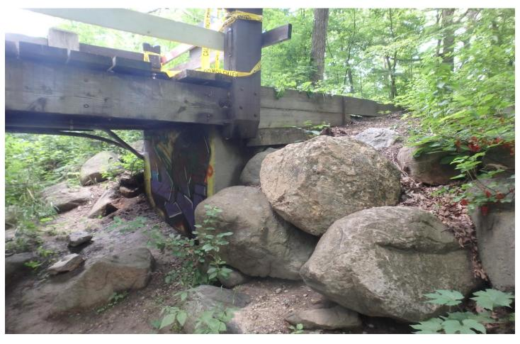
Existing Abutment & Slope Protection & Missing Approach Railing
