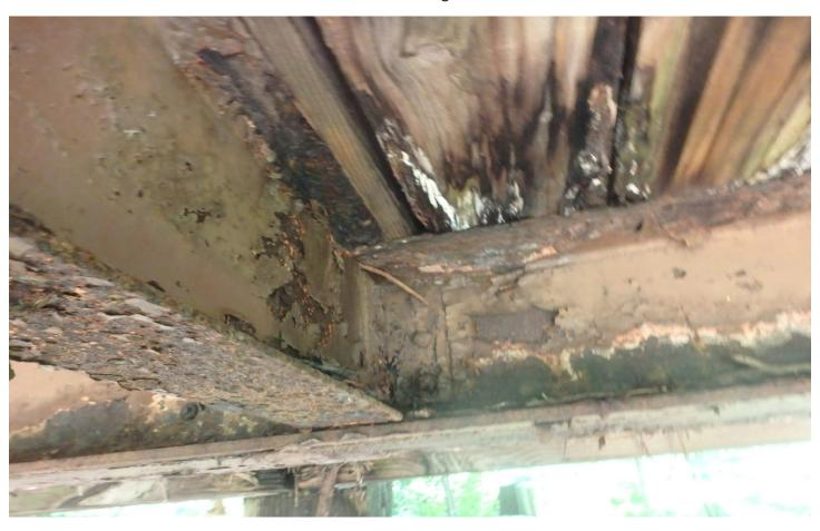
Underside of Deck showing corroded steel and rotted wood decking
