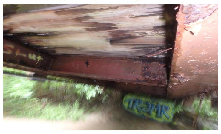
Underside showing the General Rotted Wood Deck and Corroded Supporting Structural Steel
