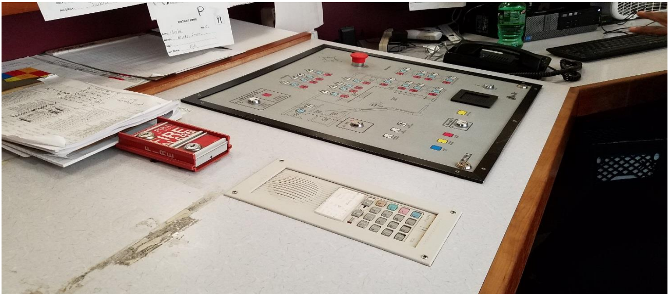
Control panel located at each JCO station inside each pod used to monitor youth in their cells.
