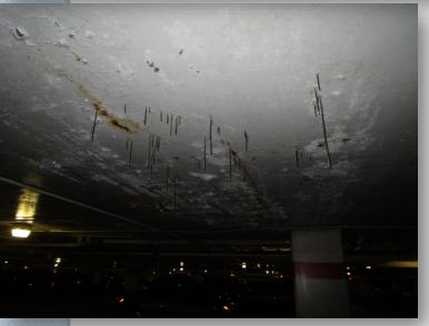
Upper Left: South Kilbourn Tunnel ceiling at voided slab, netting installed in the outline in 2010 to catch falling concrete debris.
