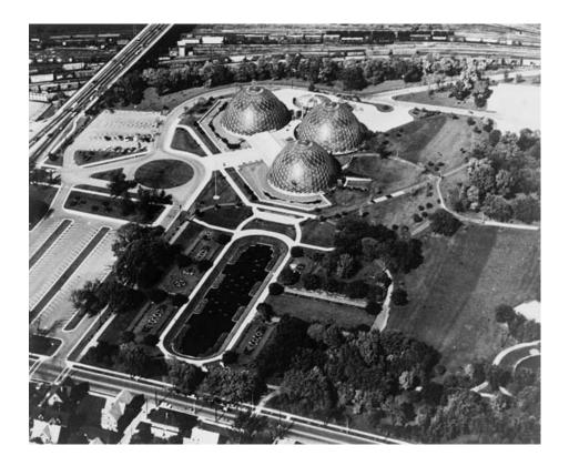
The original concrete structure was precast on site in hexagonal shapes and erected on temporary steel framing. The glazing system is composed of triangulated aluminum frames and single pane wire glass. The frames rest on the concrete structure through stainless steel posts at nodes. This late 1950's design used advanced concepts in design and state-of-the-art construction techniques.
