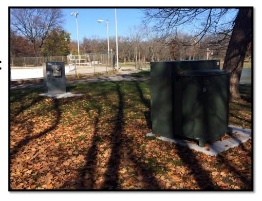
• New WE Energies electrical service to replace the outdated City of Milwaukee electrical service to the service yard, boathouse, bath house and pool. Project included removing existing electrical system components and installing new distribution and service panels, controls, junction boxes, conduit and wiring, meter pedestals and sockets, etc.
