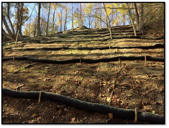
Slope stabilization to address bluff erosion damage along the Beerline segment of the Oak Leaf Trail caused by 2010 flooding
