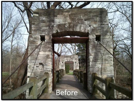
stone joints and buttresses, repointing stone joints, adding flashing to protect against water penetration, replacing steel floor beams and cross bracing, and replacing the support for the center stringer with a support that will shed water and reduce corrosion
