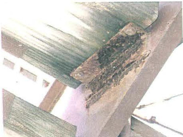
McCarty Water Slide September 2009 Steel brackets supporting the stair treads
