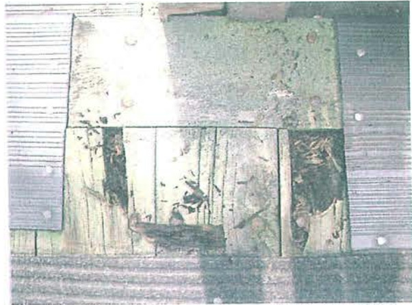
Sheridan Water Slide September 2009 Timber landings were deteriorated
