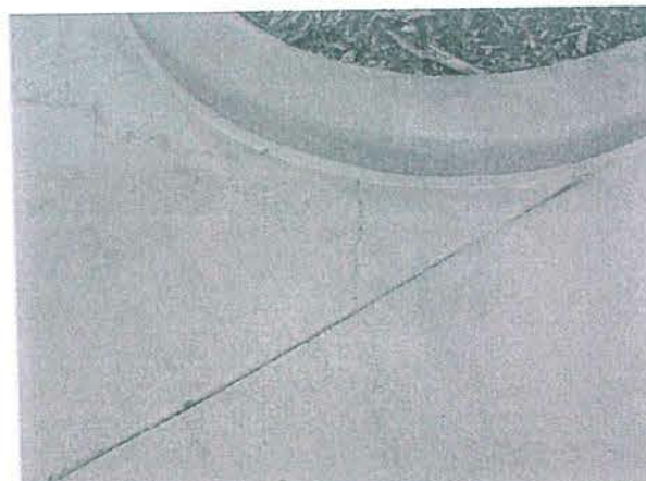
David Schultz Aquatic Center September 2009 Shrinkage cracks in new deck slabs
