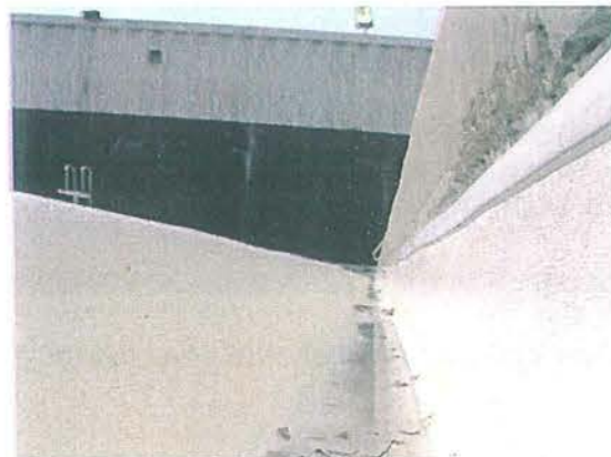
September 2009 Wilson Diving Pool Gutter - After PVC Pool Liner
