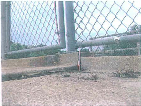
Jackson Park Swimming Pool September 2008 Deck slabs out of level
