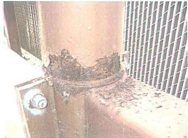
Sheridan Water Slide September 2009 Steelwork needs blasting and protective coatings
