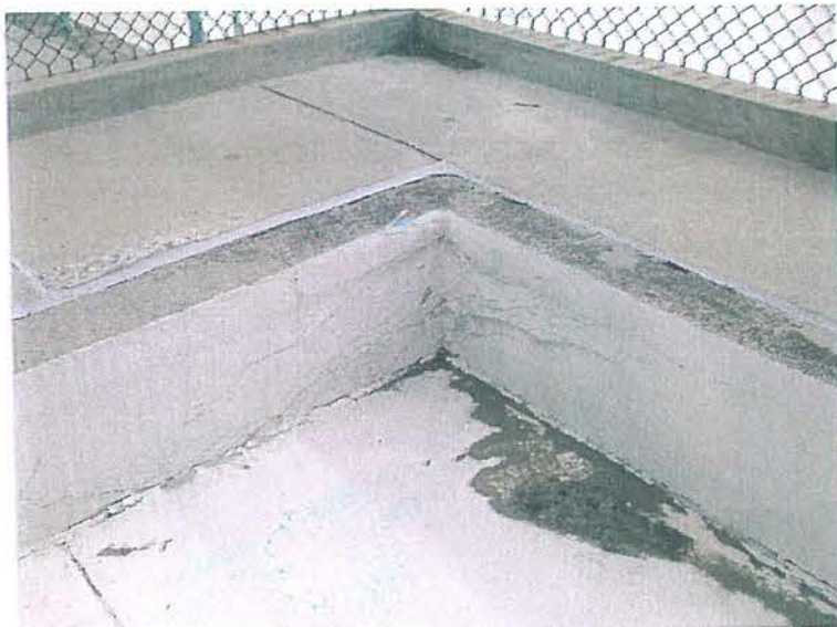
Sheridan Park Wading Pool - Wall cracking at corner September 2009
