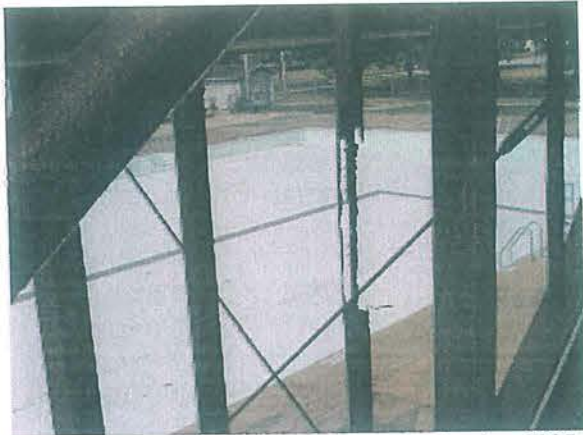
McCarty Water Slide Baluster rusted through
