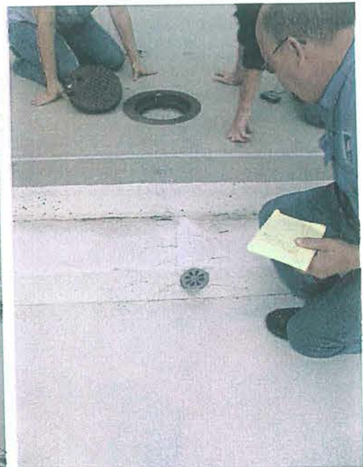
Step heaving at Inlet
