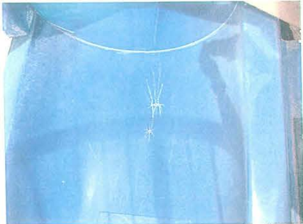
Sheridan Water Slide September 2009 Slide flume has minor spider cracking
