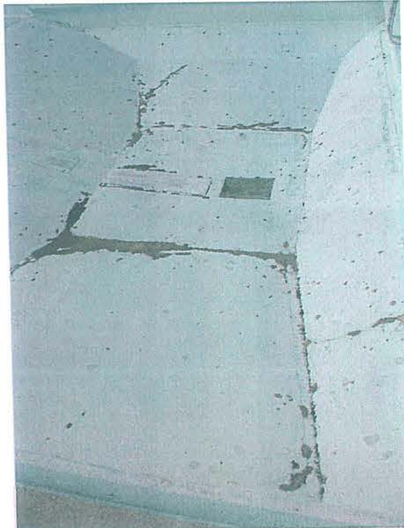
Grobschmidt (Oak Creek) Swimming Pool September 2009 Diving Well – note extensive patching and caulking of deteriorated slabs.
