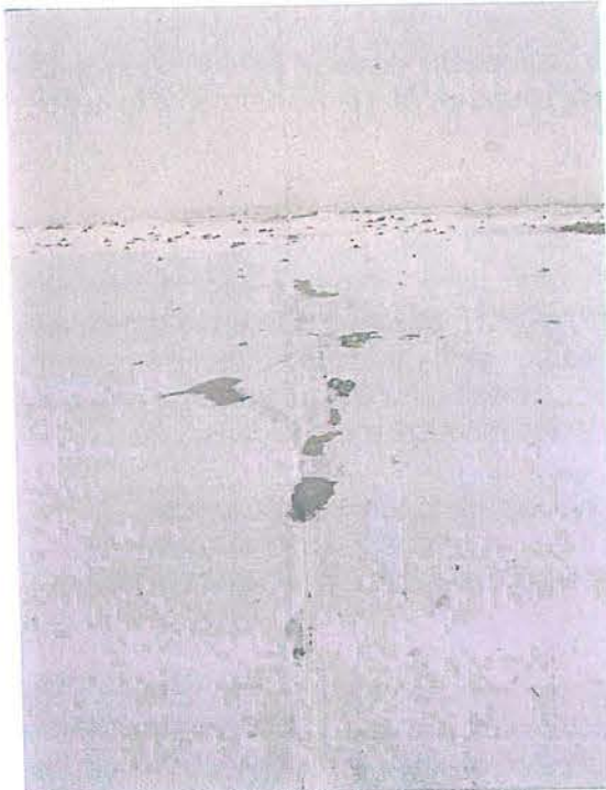
Holler Swimming Pool - Spalls, failed patches, and deteriorated slab edges
