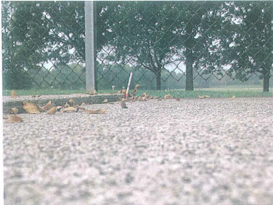
Hales Corners Swimming Pool Pool Deck – note out of level concrete slabs
