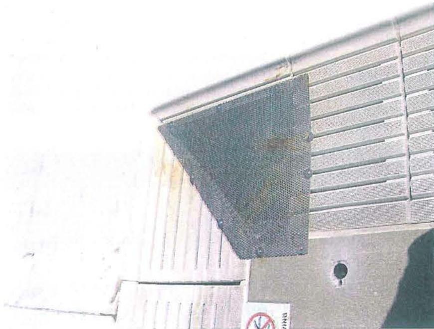
Cool Waters Aquatic Center Precast Pool Coping Stones – temporary corner piece
