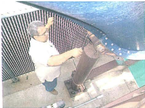
Sheridan Water Slide September 2009 Steel columns are rusting, but are structurally sound
