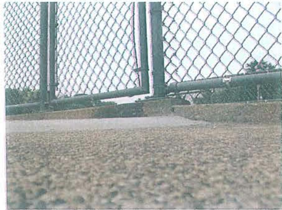
Jackson Park Swimming Pool September 2009 Out of level deck slabs with transition
