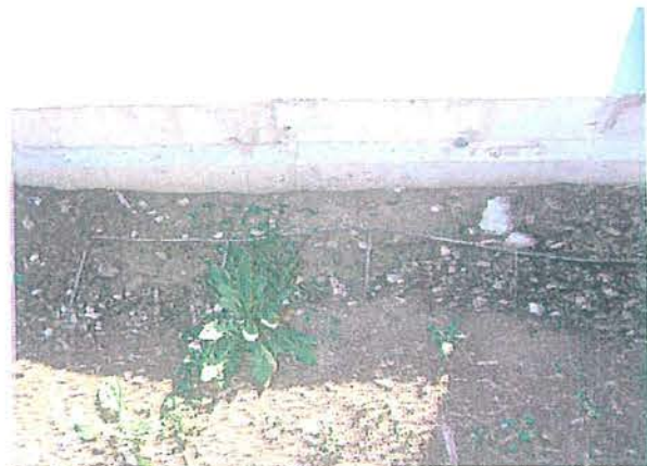
David Schultz Aquatic Center September 2010 Grounding wires exposed behind pool wall where slides enter pool
