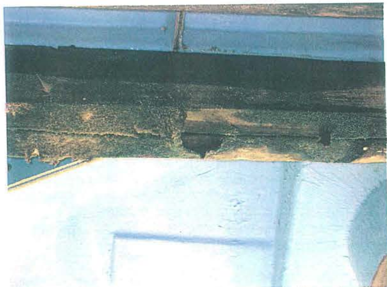
Cool Waters September 2009 Moss growing on timber structural members
