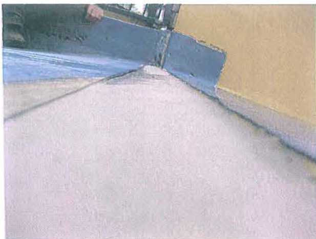
Cool Waters Aquatic Center May 2010 Tot Slide Entry Well to Flume Delaminating fiberglass
