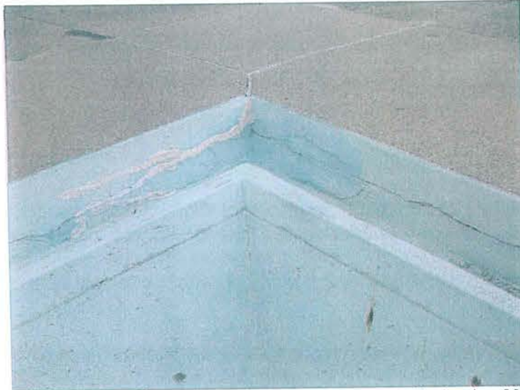
Grobschmidt (Oak Creek) Swimming Pool September 2009 Scum Gutter NW Corner shallow area – note long crack in gutter back wall
