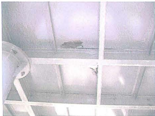
David Schultz Aquatic Center September 2010 Protective Coatings failing below slide tower landings
