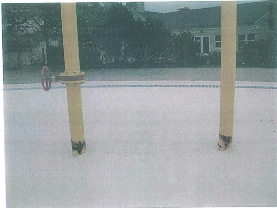
Cool Waters Aquatic Center Note rusting at base of pool toys
