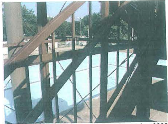
McCarty Water Slide Repaired Baluster (new baluster is rusting because protective coatings were not applied)
