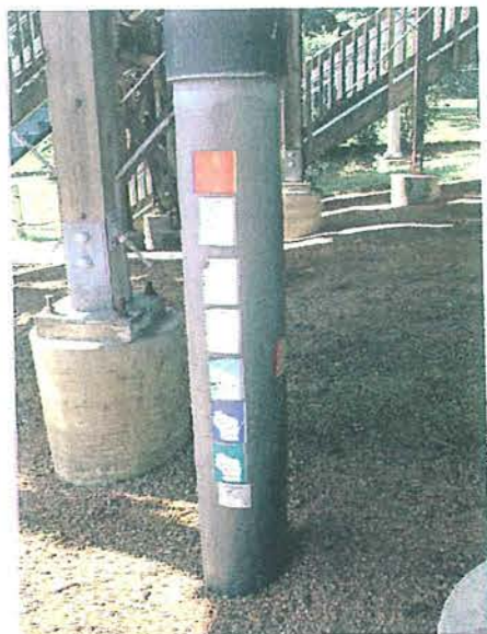
Cool Waters September 2009 Concrete Footings – no cracks or other damage
