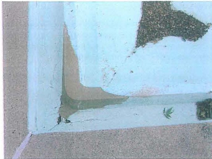
Grobschmidt (Oak Creek) Swimming Pool September 2010 SW corner deep area Repaired concrete gutter lip
