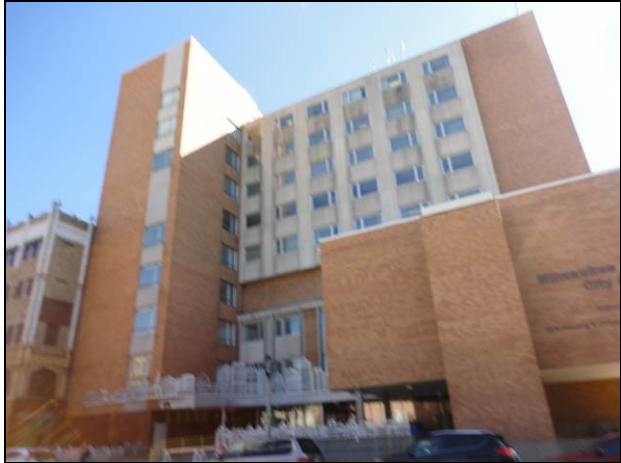
9-Story Building Exterior
