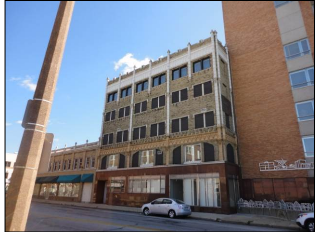
5-Story Building Exterior
