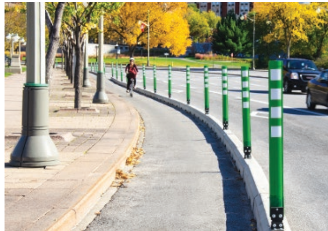
Pre-cast or cast-in-place concrete curb
