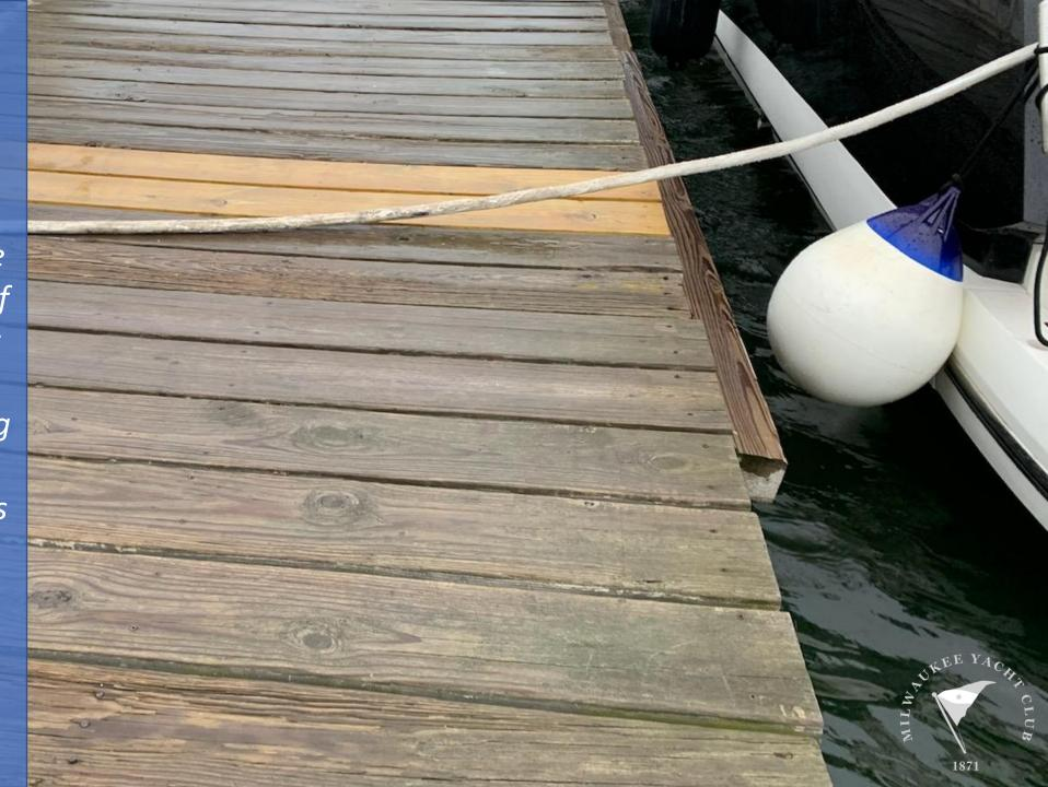
Notwithstanding the repair issues, the current docks are a fixed structure. Fixed piers become problematic when the water level varies especially during extremes (i.e., high/low water cycles, storms, ice).
