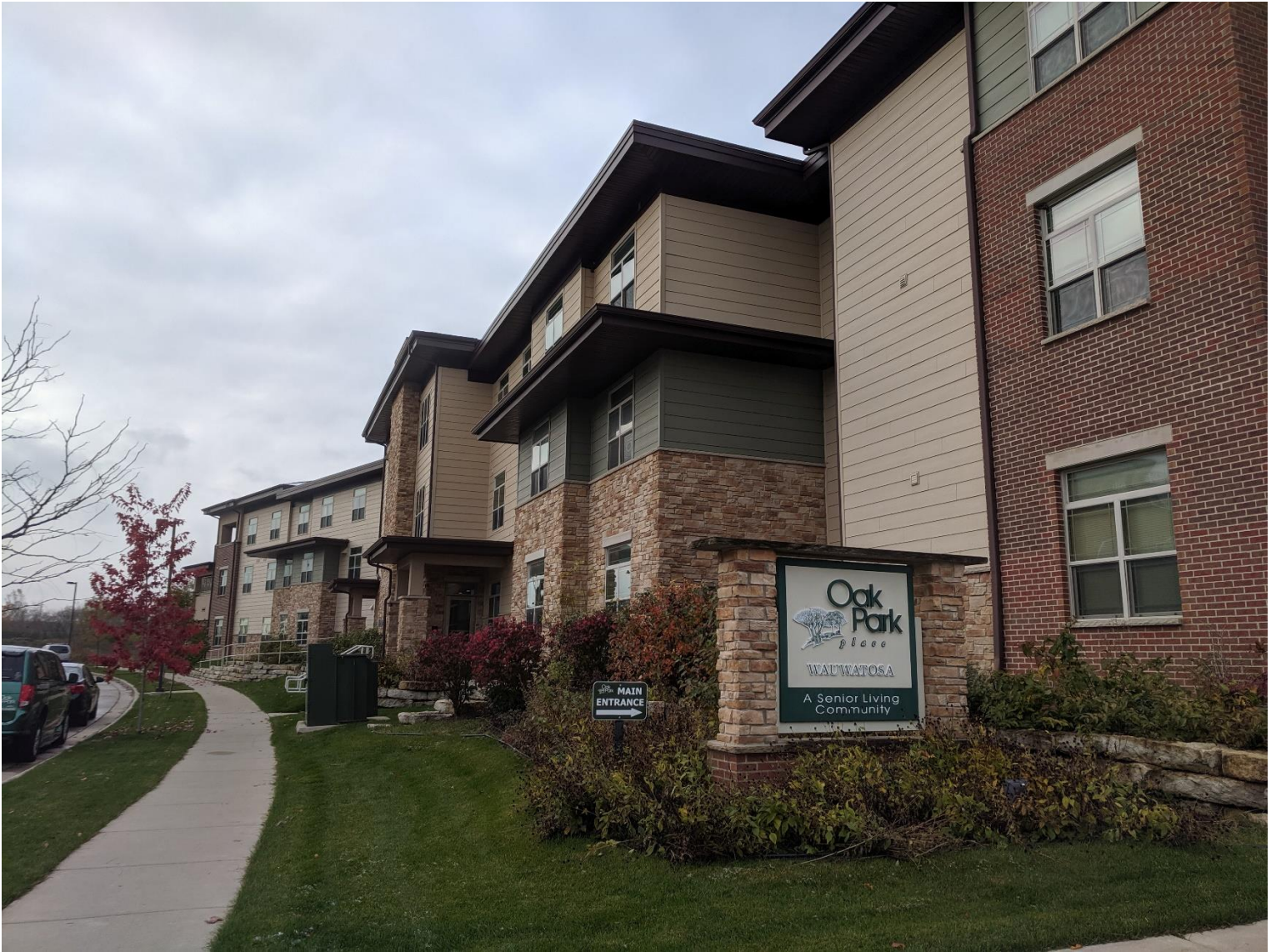
Existing Use – Oak Park Place (1621 Rivers Bend) – Fall 2019
