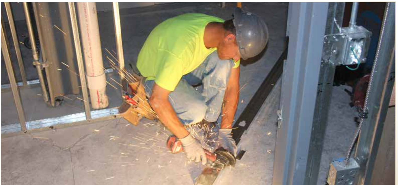
Worker cutting metal on McKinley Center Project.
