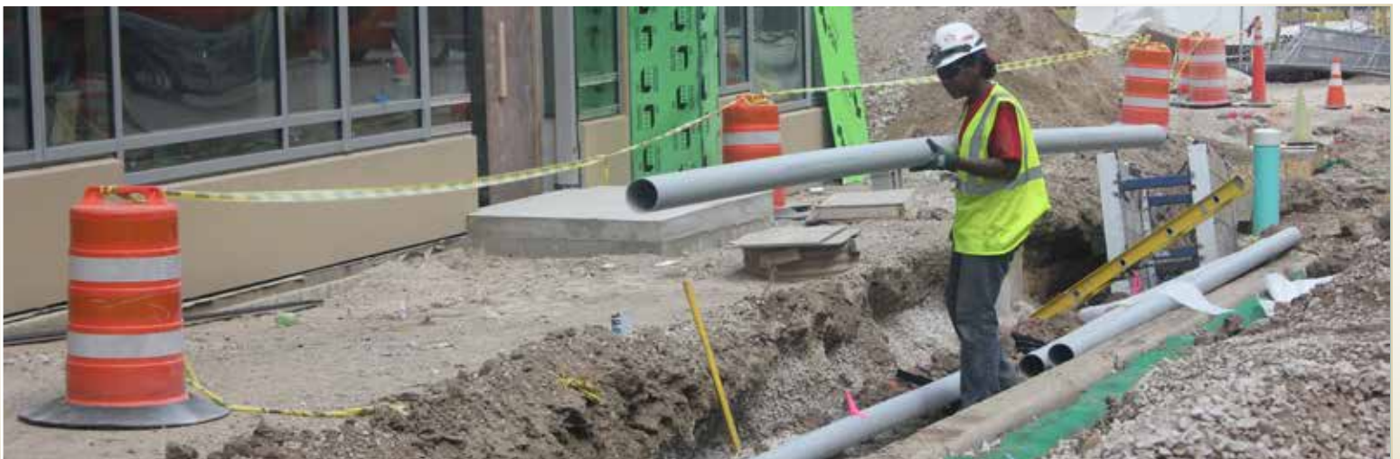
Electrician carrying piping to 5th Street Parking Structure.
