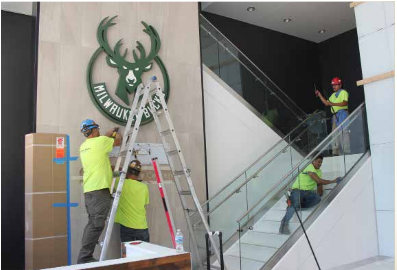
Workers completing final construction on F & MCW Sports Science Center project.
