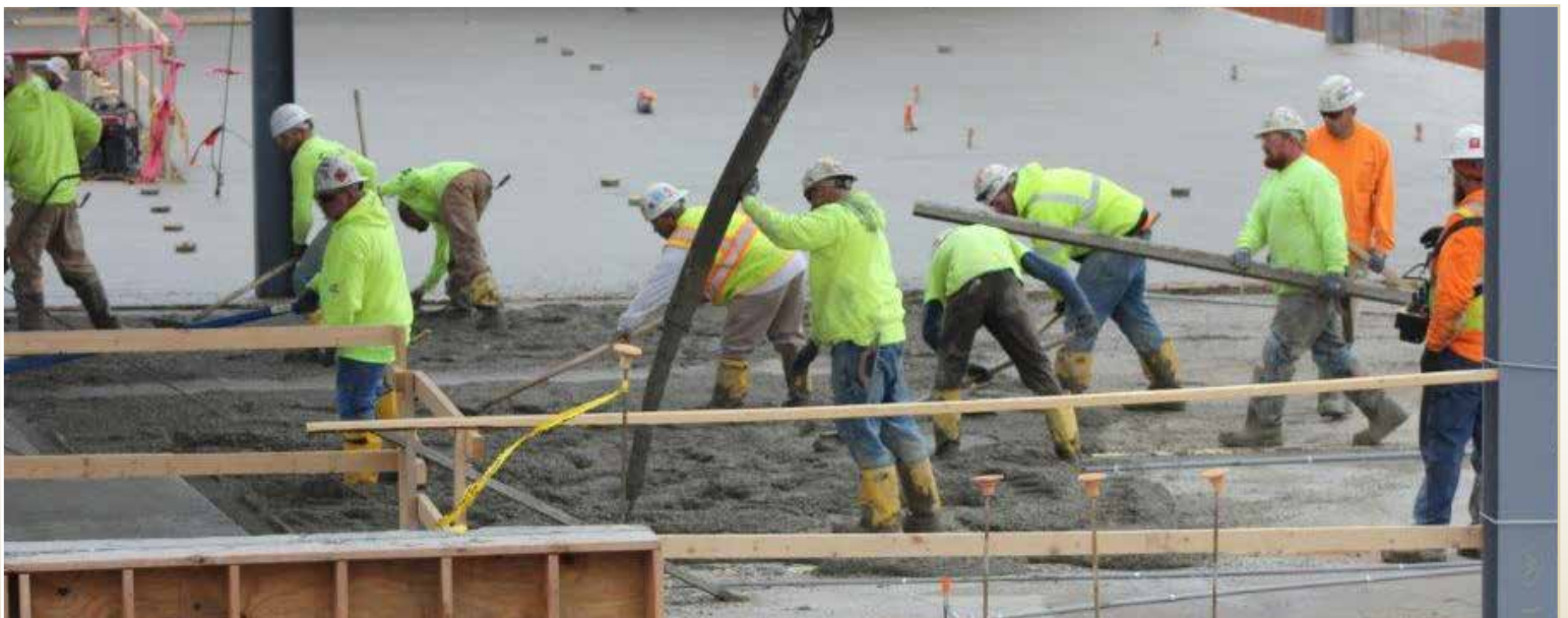
Workers laying concrete on 5th Street Parking Structure.
