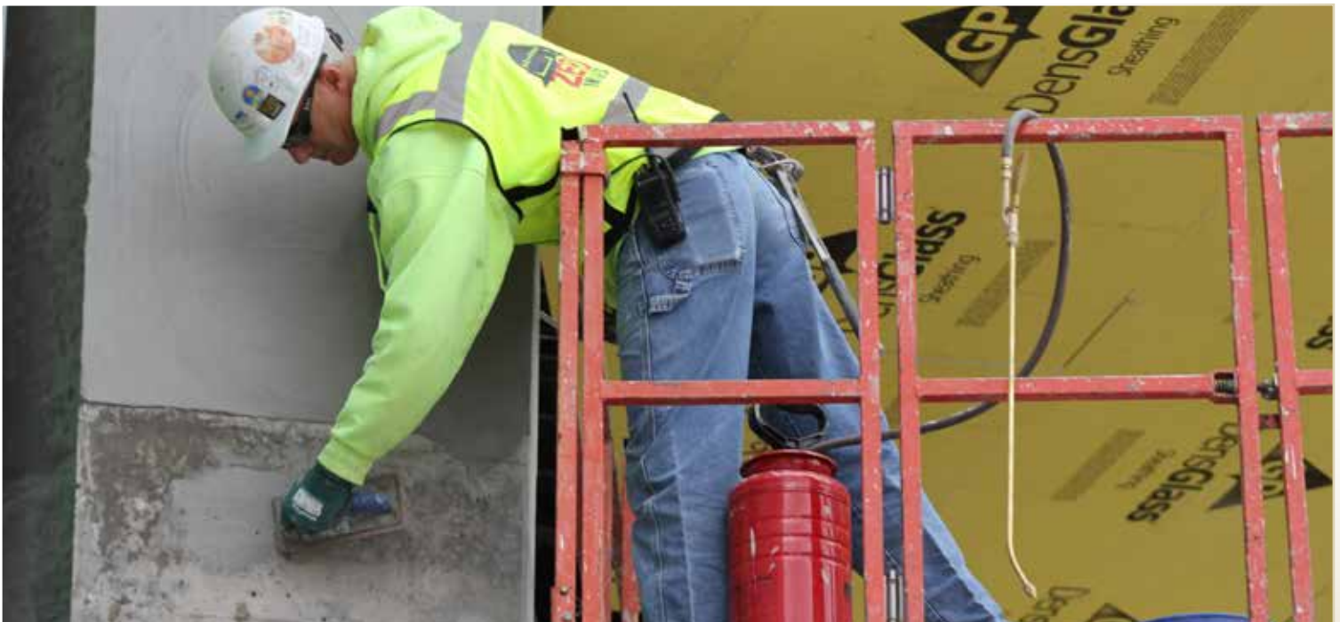
Laborer working on project site.
