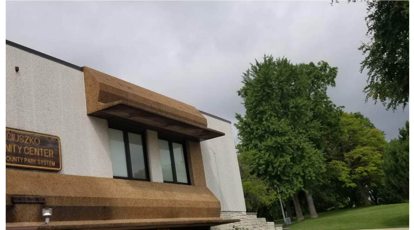
Photo 2: Precast Panel Cracking
