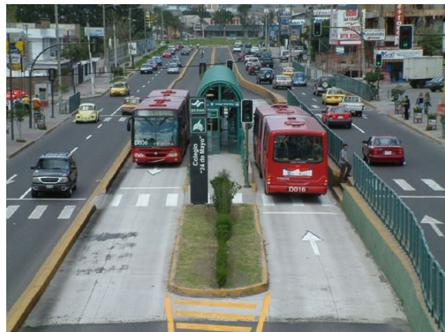
The running ways for Mexico City’s BRT system are dedicated median lanes. Physical barriers prevent other traffic from entering bus lanes.
