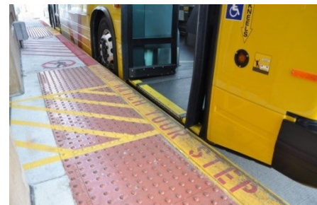
A BRT service in Minneapolis features level boarding at bus stops.
