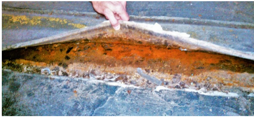
An expansion joint was so loose it could be physically lifted.
