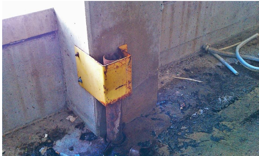
An expansion joint was so loose it could be physically lifted.
