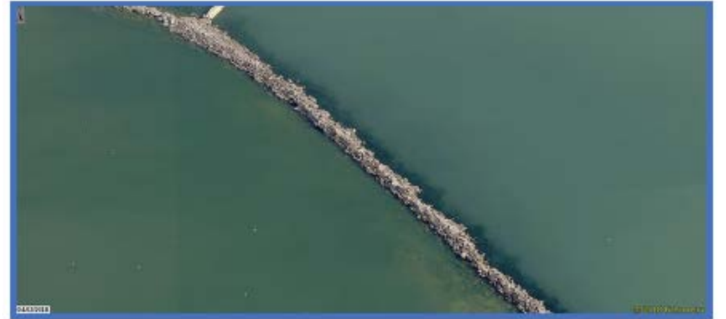
South Shore Breakwater – Image Captured May 2018, Source: MCLIO
