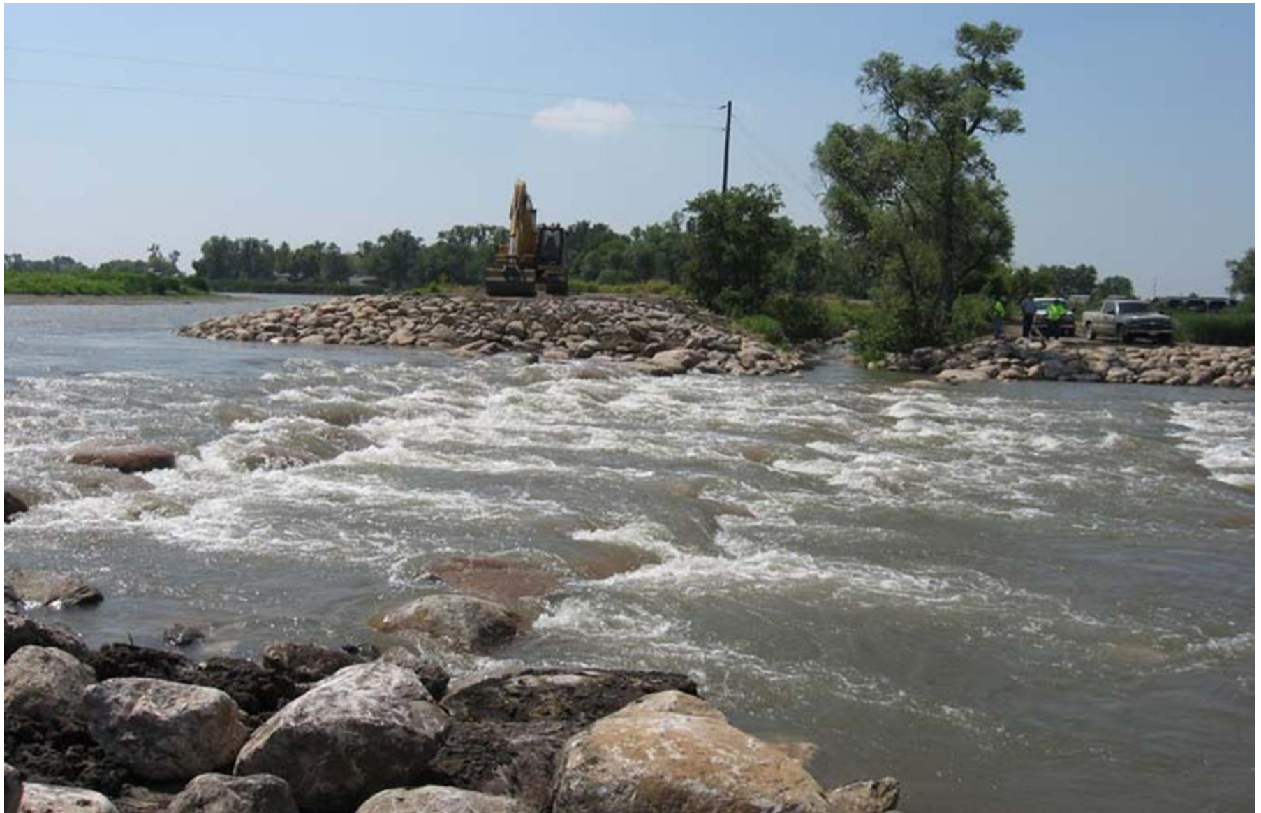
Figure 91. Rapids replacing dam to provide grade control and facilitate fish and canoe passage. Reconnecting Rivers: Natural Channel Design in Dam Removals and Fish Passage , p. 80. Minnesota Department of Natural Resources Ecological Resources Division, 2010.
