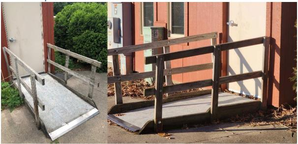
As you can see by the picture above the ramp is a man-made structure that was put together as a temporary fix. This temporary fix has been at the County for my entirety, which is over 10 years. The slope of the ramp, and handrails are not ADA compliant, and do not meet the ADA Standards. The estimated repair costs for this is estimated at \$14,953. There are additional areas of asphalt that Parks is looking at
