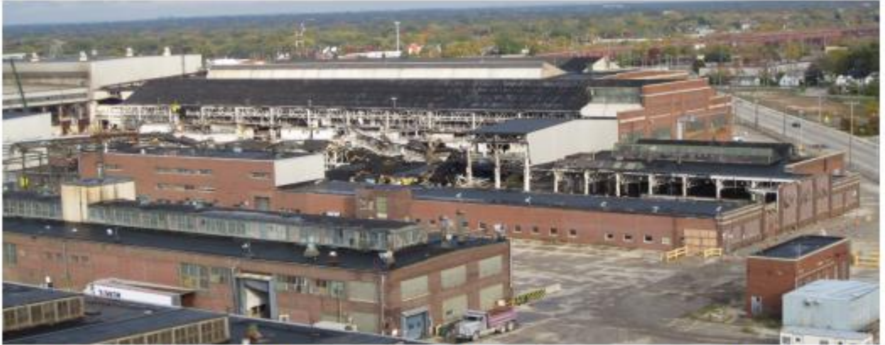
Former Tower/ A.O. Smith site in October 2009. Note Building 37 (center) is collapsing. (City of Milwaukee)
