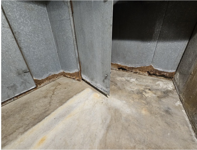
Photo 7: HVAC Corrosion
