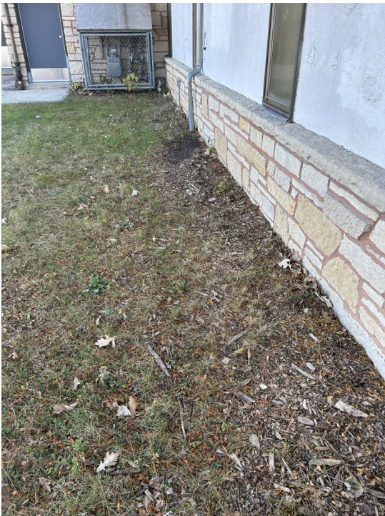
Photo 3: Unpaved area adjacent to north side of building.
