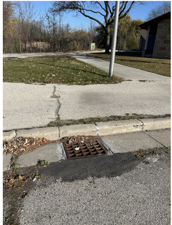
Photo 12: Exterior of inlet from Photo 10.
