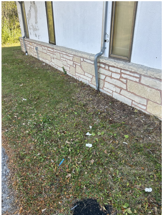
Photo 4: Unpaved area adjacent to north side of building.
