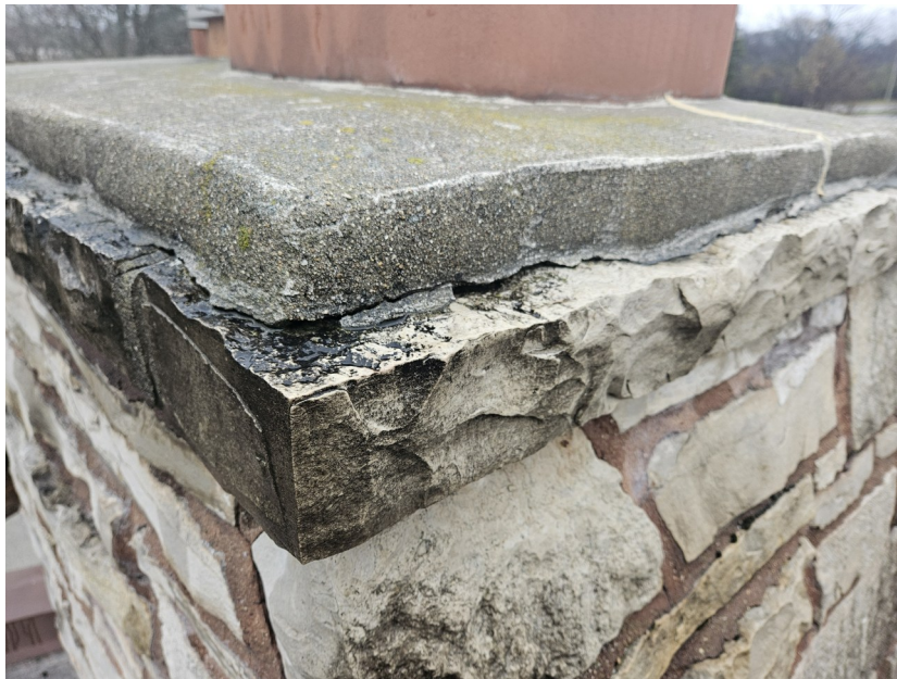
Photo 16: Cracking Mortar
