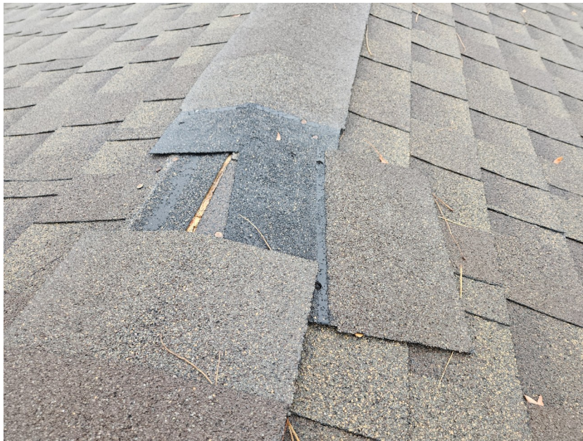
Photo 10: Roof Damage
