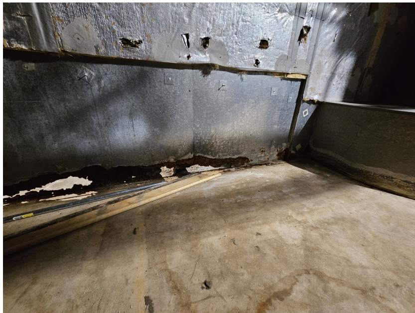
Photo 8: HVAC Corrosion
