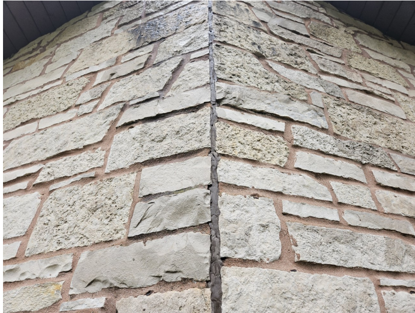
Photo 15: Failing Sealant
