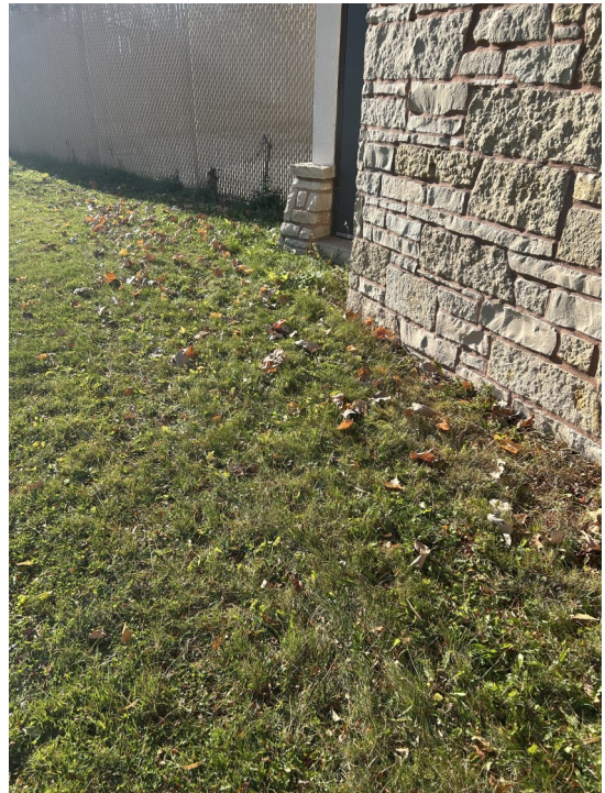
Photo 6: Unpaved area adjacent to northeast side of building.
