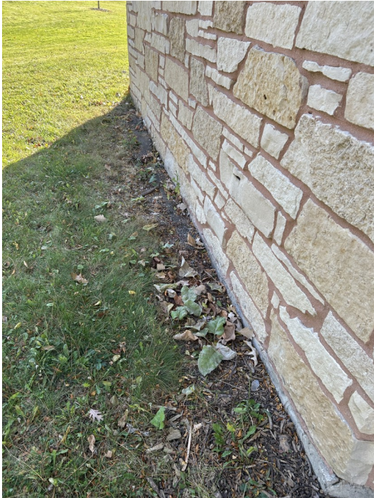
Photo 5: Unpaved area adjacent to north side of building.
