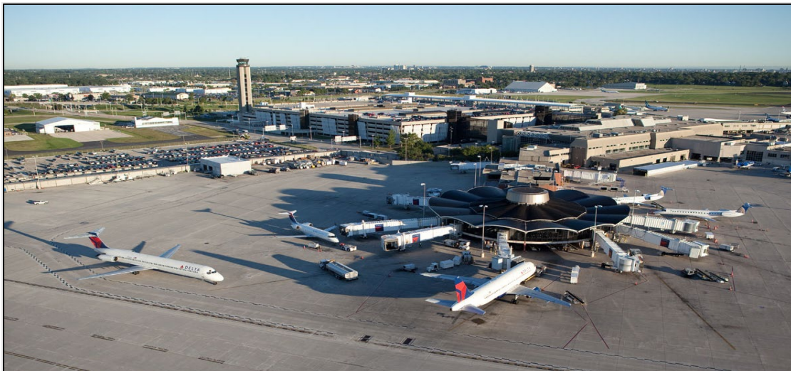
File No. 17-716: The present Concourse E, to be redeveloped as the new international terminal
