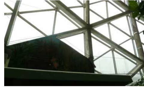
Netting for Structural Debris
