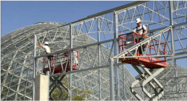
2014 Building Greenhouse Annex
