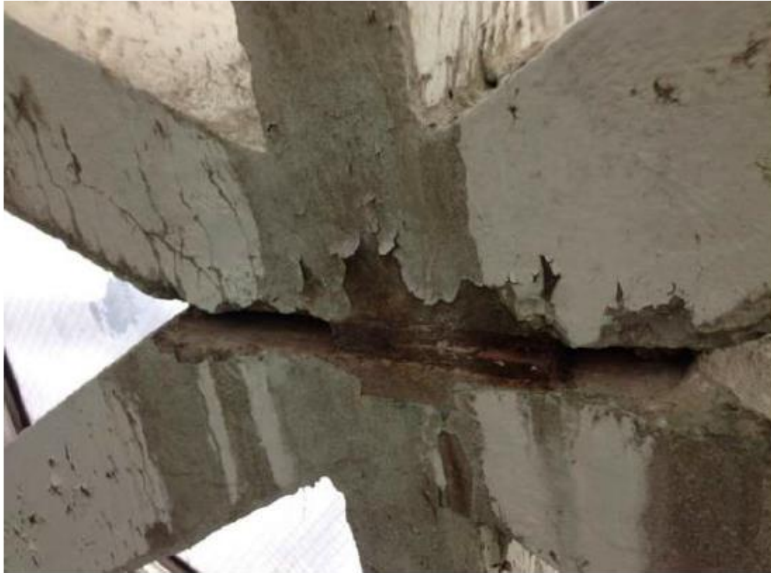
Photo F07: REMOVAL OF GROUT MAKES ROOM FOR NEW GROUT REPAIR. CONNECTION PLATE EXHIBITS SOME RUST.
