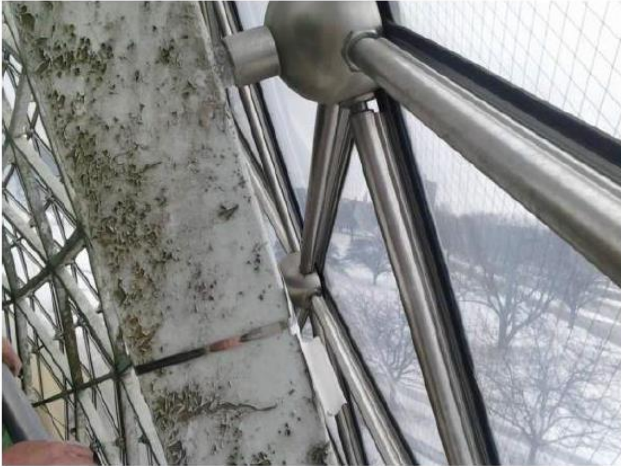
Photo F12: WATER DIVERTER INSTALLED BELOW HUB.
