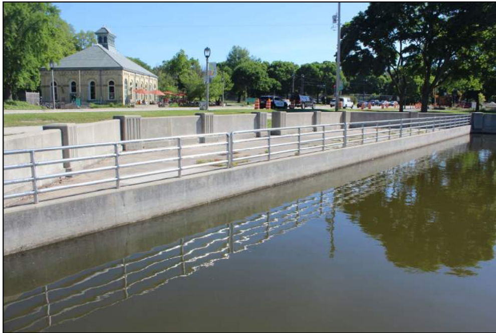
Photo 9 – View of the intake structure at the end of the Flushing Channel.
