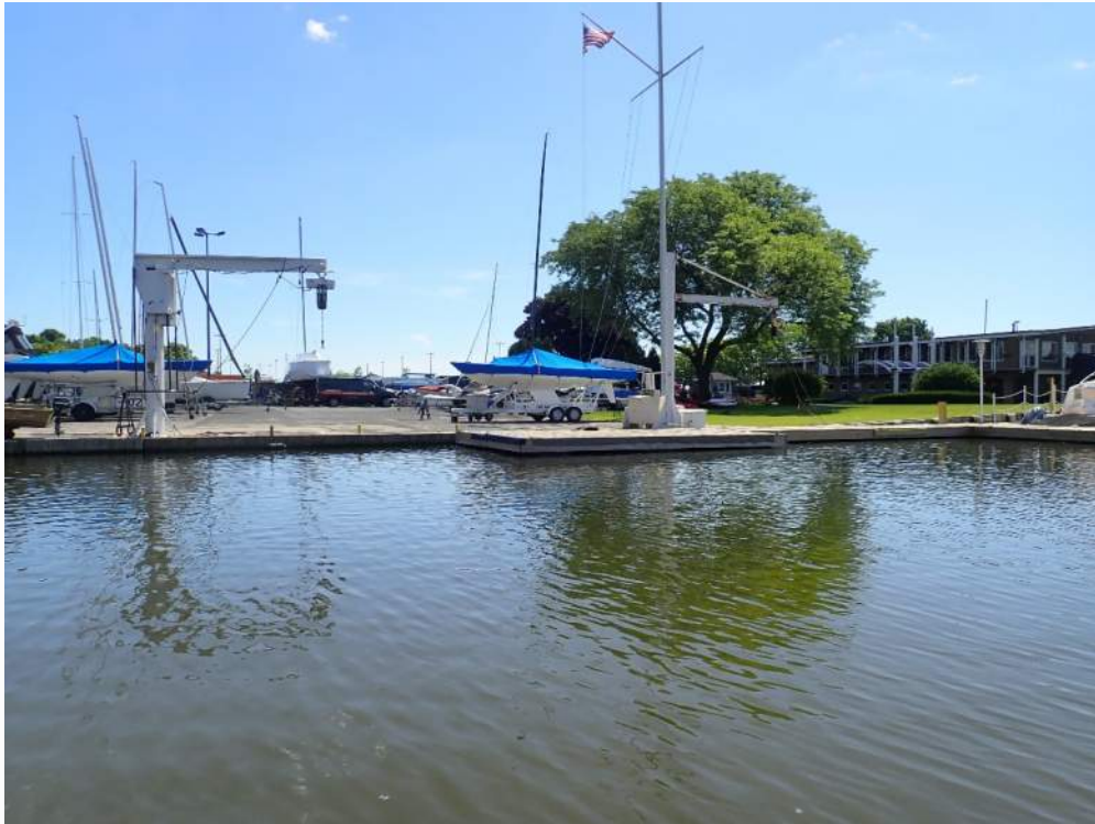
Photograph 7: View of East-Central and South-Central Flushing Channel Walls, looking east.
