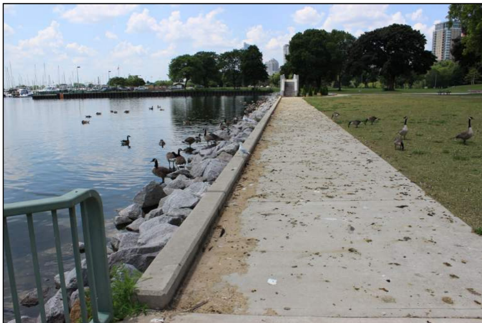
Photo 22 – Existing stone revetment that abuts the channel to the west.
