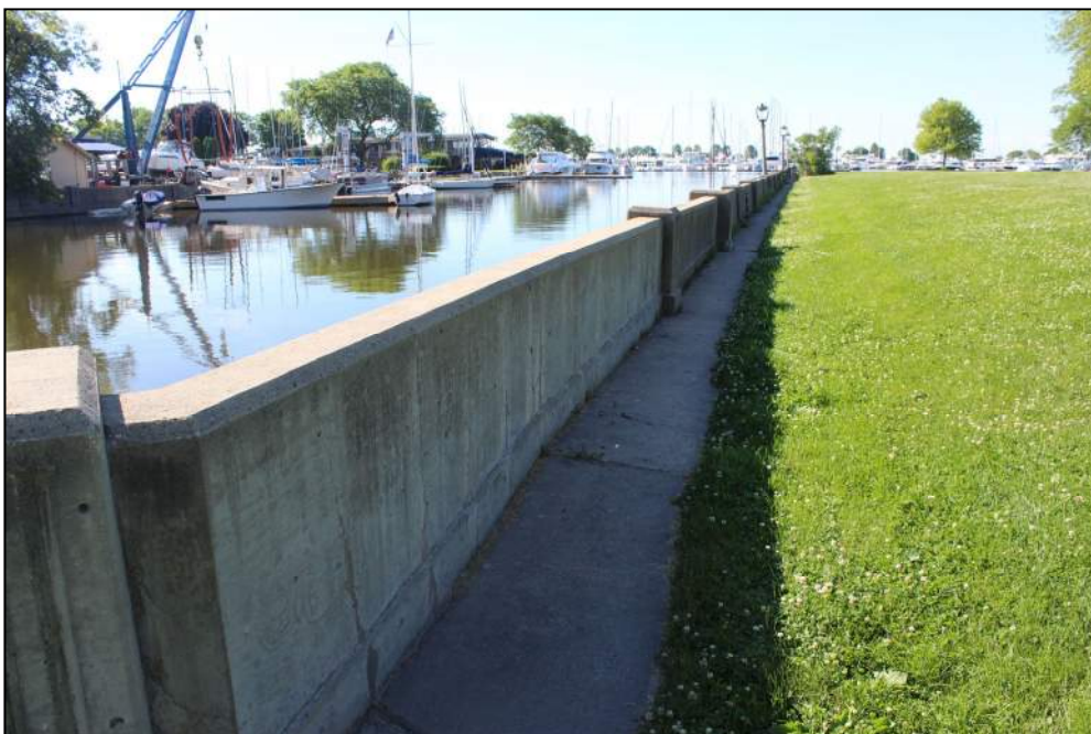
Photo 2 – View of the west channel wall facing south.
