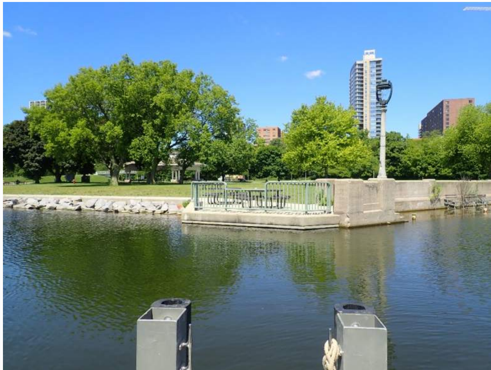
Photograph 2: View of overlook at the southwest corner of Flushing Channel, looking northwest.
