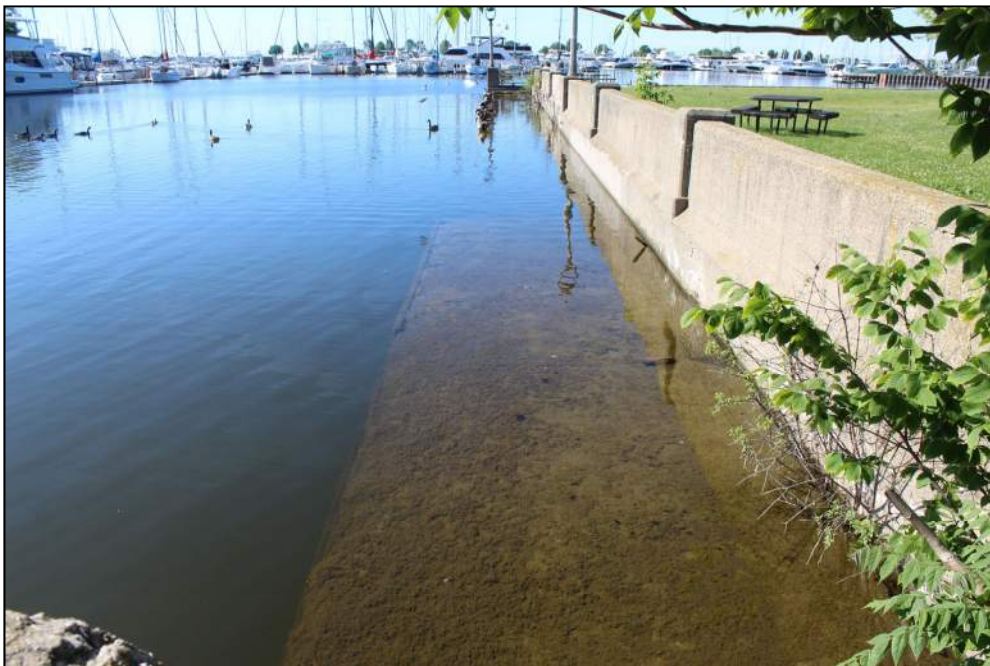
Photo 6 – Existing submerged boat ramp facing south.
