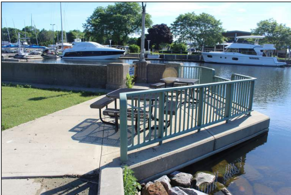
Photo 8 – View of the recently installed concrete promenade at the southeast corner of the channel.
