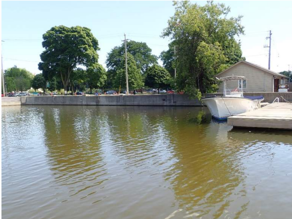
Photograph 5: View of Northeast Flushing Channel Wall (Wall Section 4), looking east.
