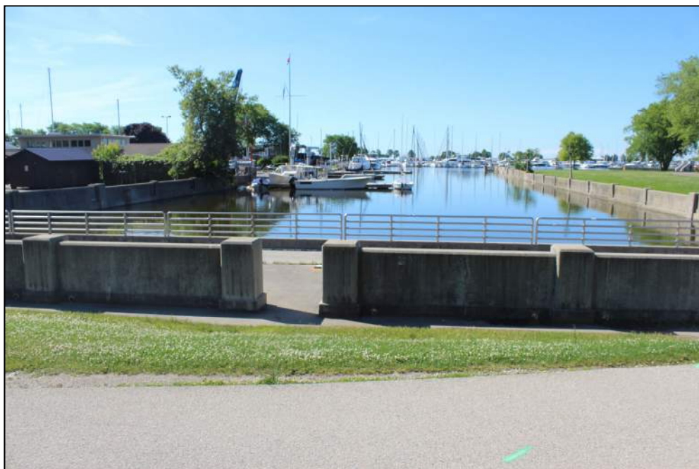
Photo 10 – View of the Flushing Channel from the intake structure facing south.
