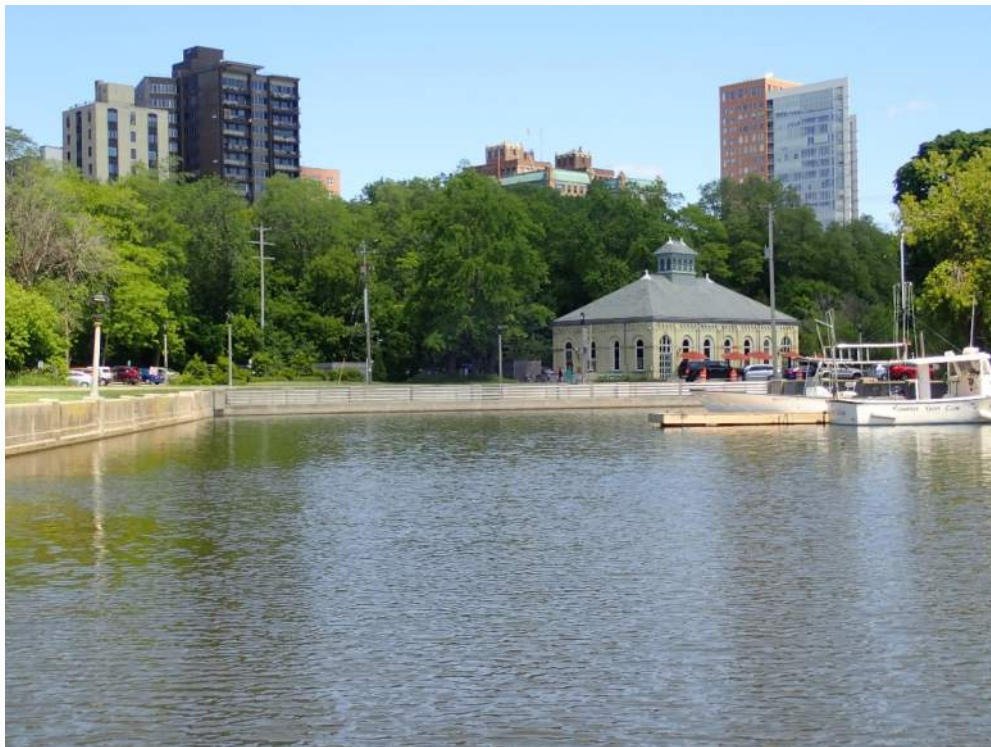
Photograph 4: View of North Wall of Flushing Channel (Wall Section 3), looking north.
