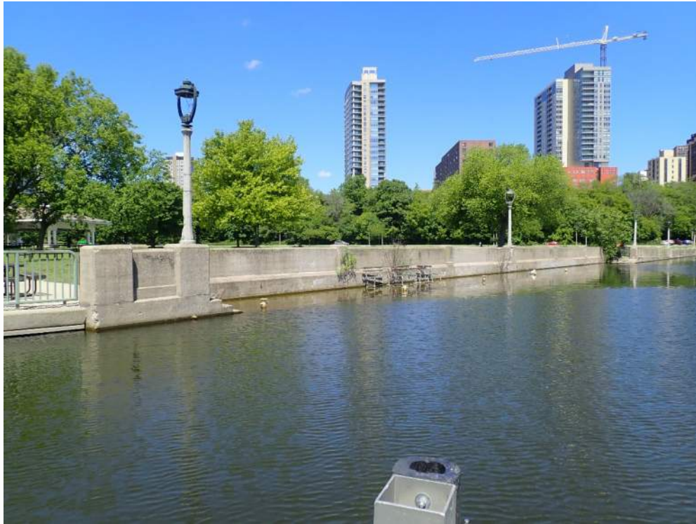
Photograph 3: View of west wall of Flushing Channel (Wall Section 2), looking northwest.
