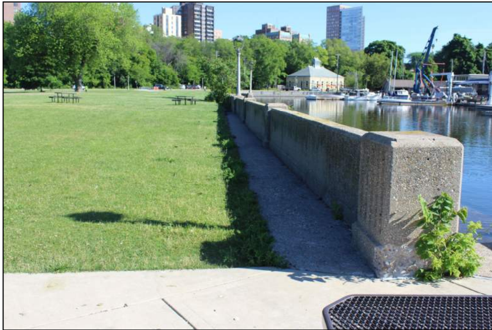
Photo 7 – View of the west channel wall facing north.
