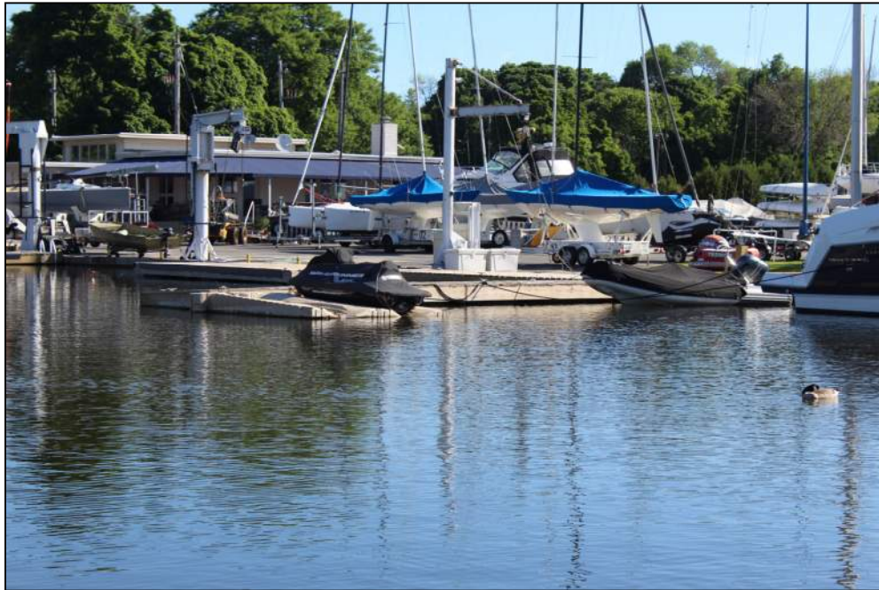
Photo 15 – View of the east channel wall with floating docks and davits, facing northeast.
