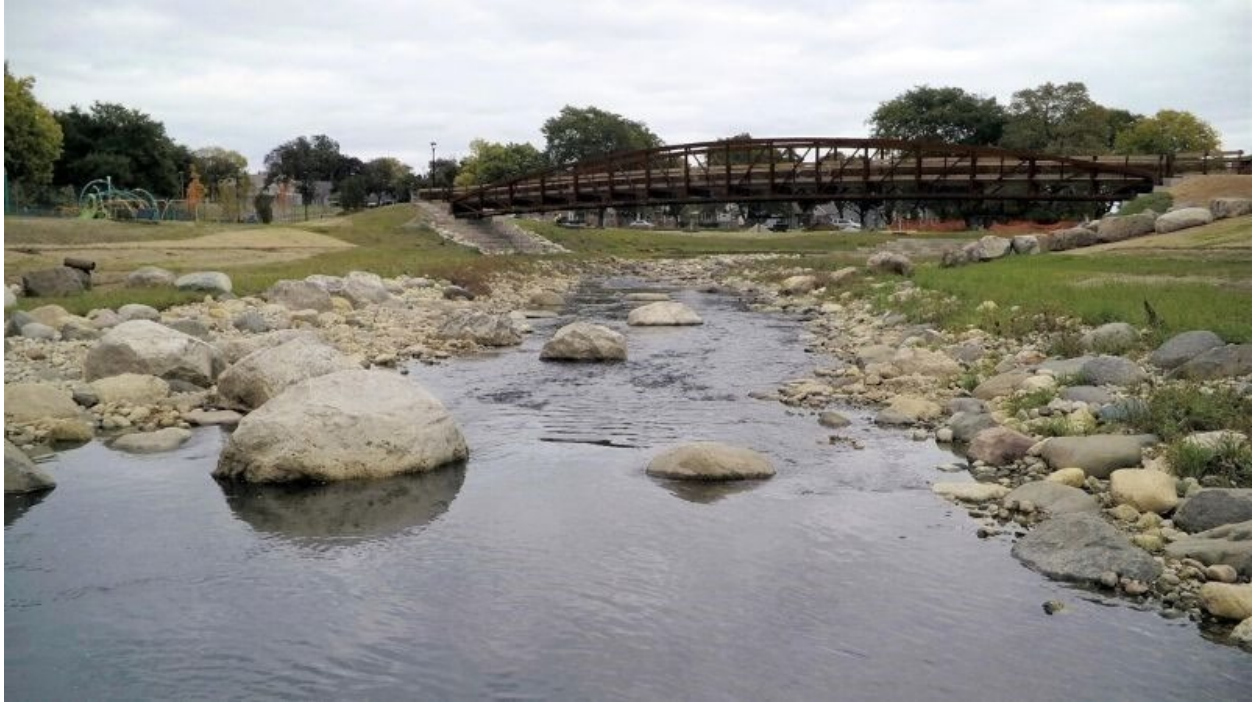
Image above: Kinnickinnic River in Pulaski Milwaukee Park after removal of concrete channel
