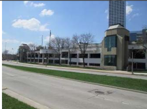
Exterior View of Parking Structure
