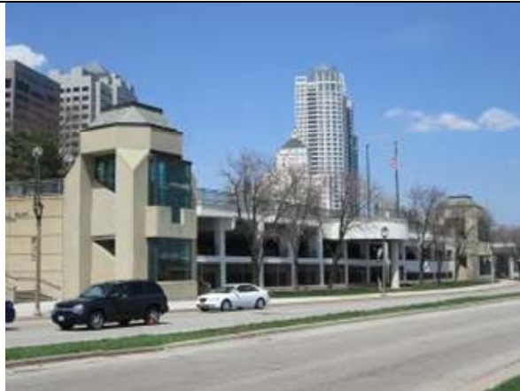
Exterior View of Parking Structure
