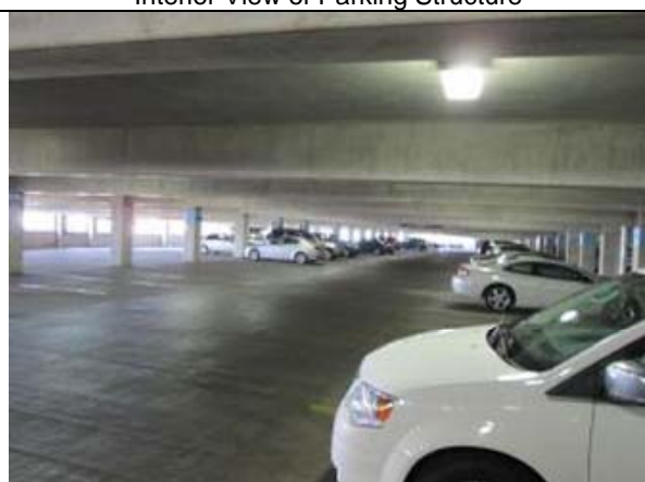
Interior View of Parking Structure
