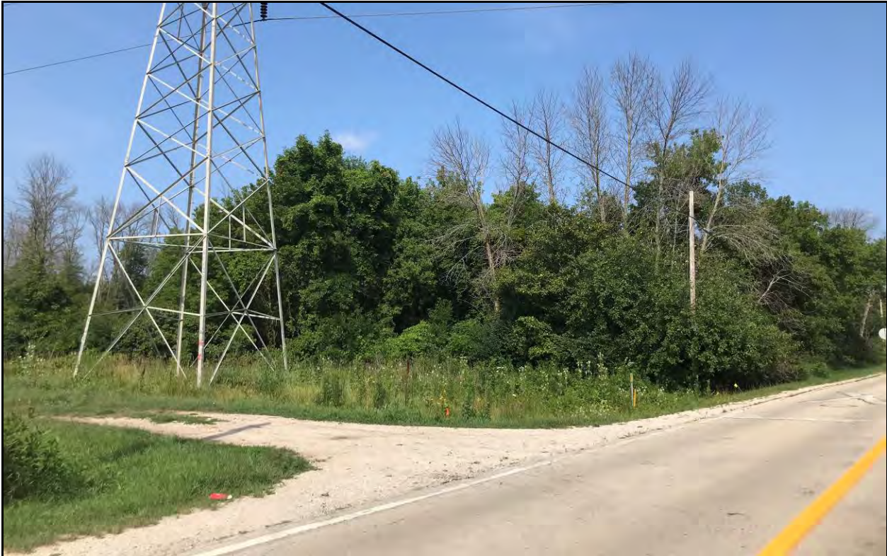
Representative photograph of the subject property looking northeast from East Forest Hill Avenue.
