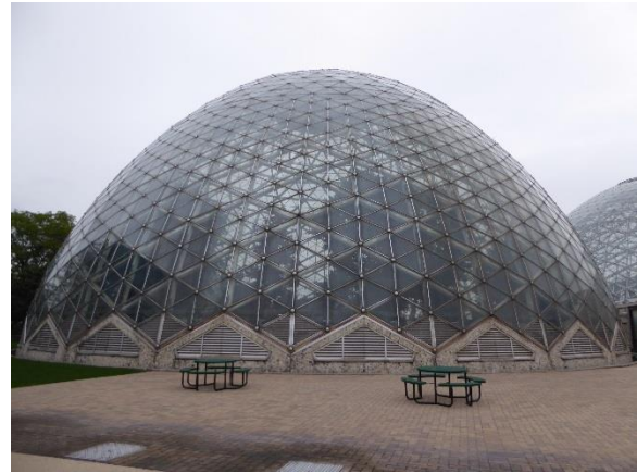
Figure 2. View of the Show Dome
