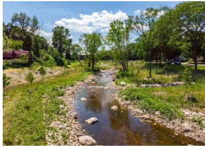
Figure 6.24 Example of Creek Restoration Along Underwood Creek
