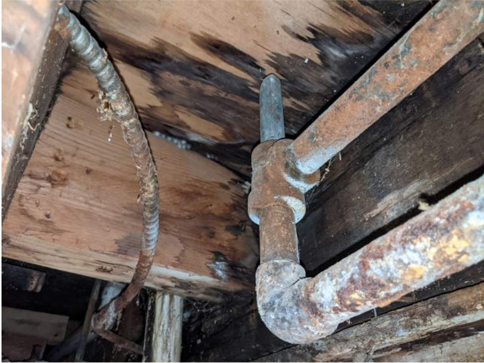
Photograph 3: Sheathing Deterioration
