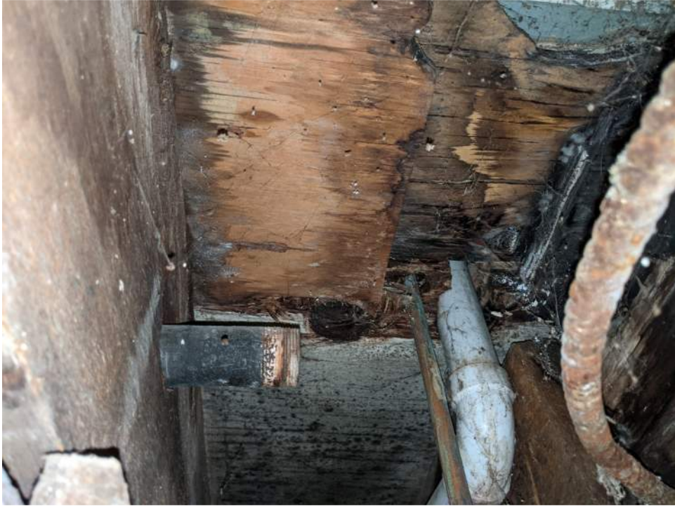
Photograph 1: Sheathing Deterioration
