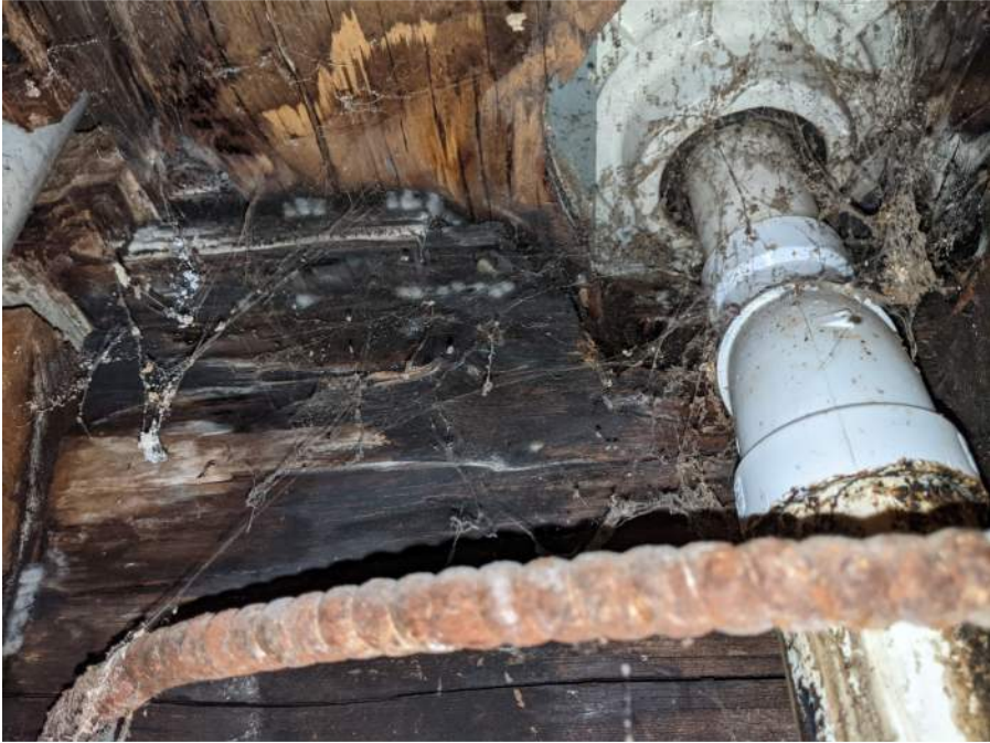
Photograph 5: Sheathing Deterioration
