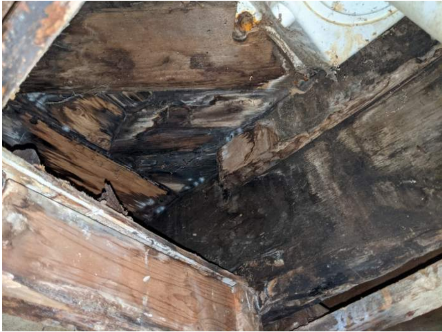
Photograph 4: Sheathing Deterioration
