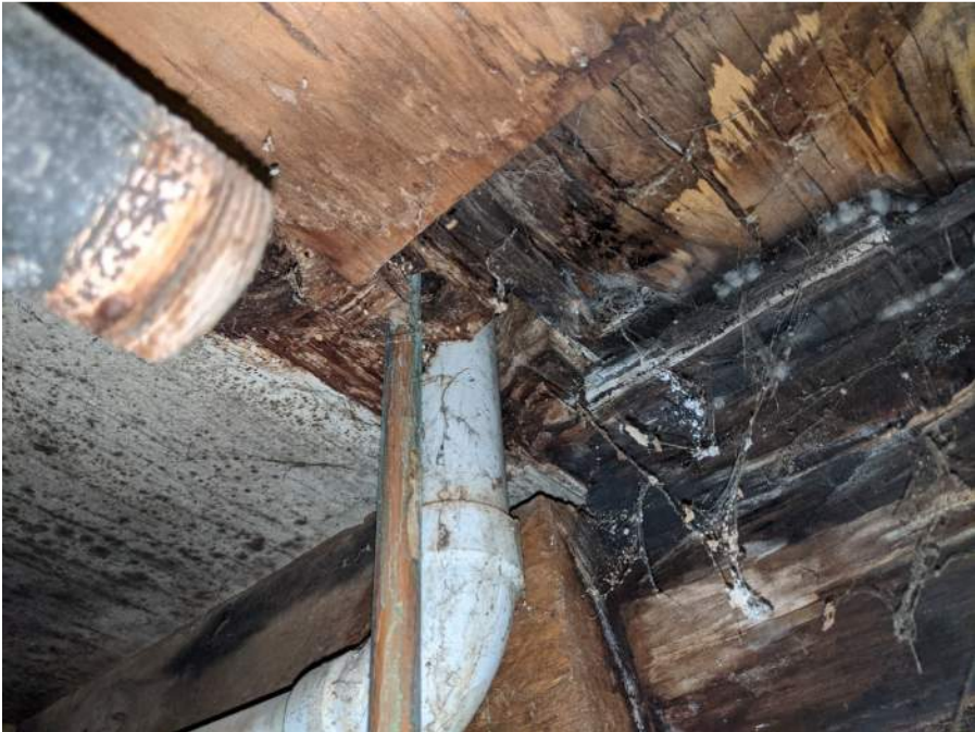
Photograph 6: Sheathing Deterioration
