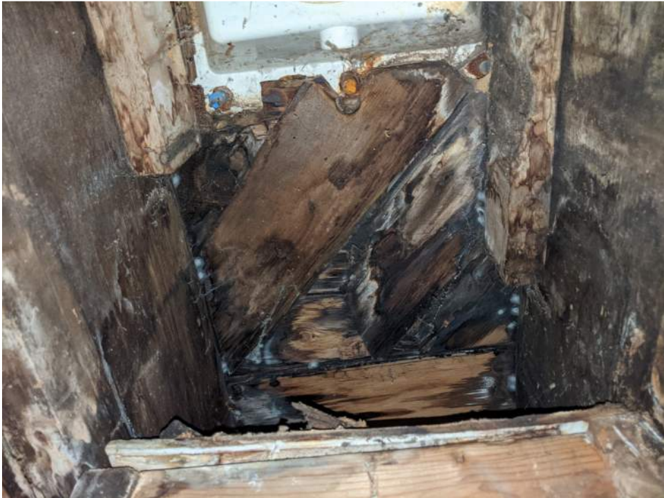
Photograph 2: Sheathing Deterioration
