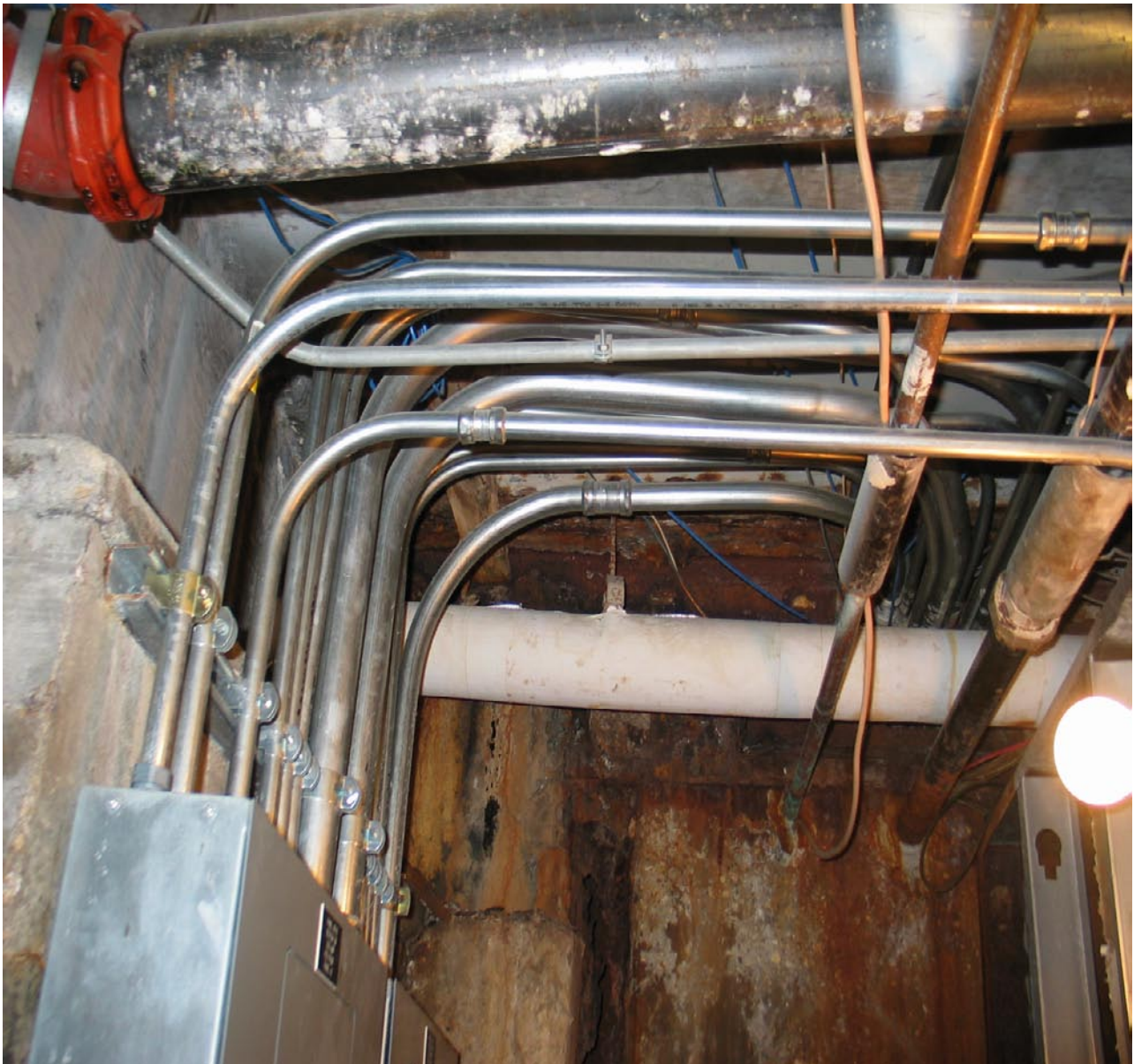
Walls on the lower level of museum have severe surface deterioration near the lunchroom area.
