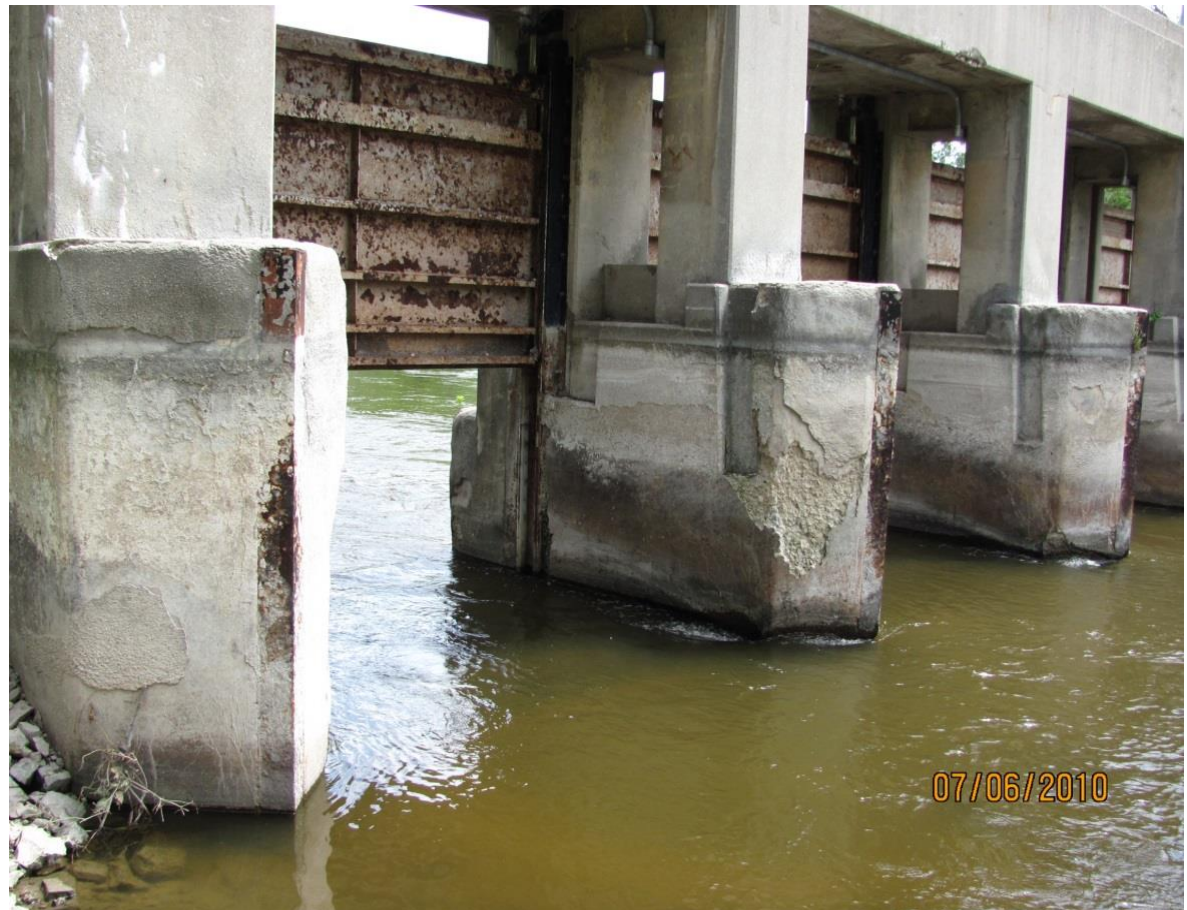
Photo 3: Upstream side of Pier 1 (left), Pier 2 (center), and Pier 3 (right) in 2010
