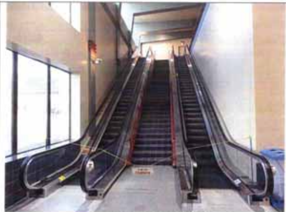
Escalators to Second Floor
