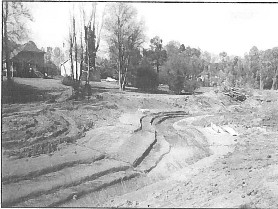
Photograph 1. Soil fabric lifts under construction.
