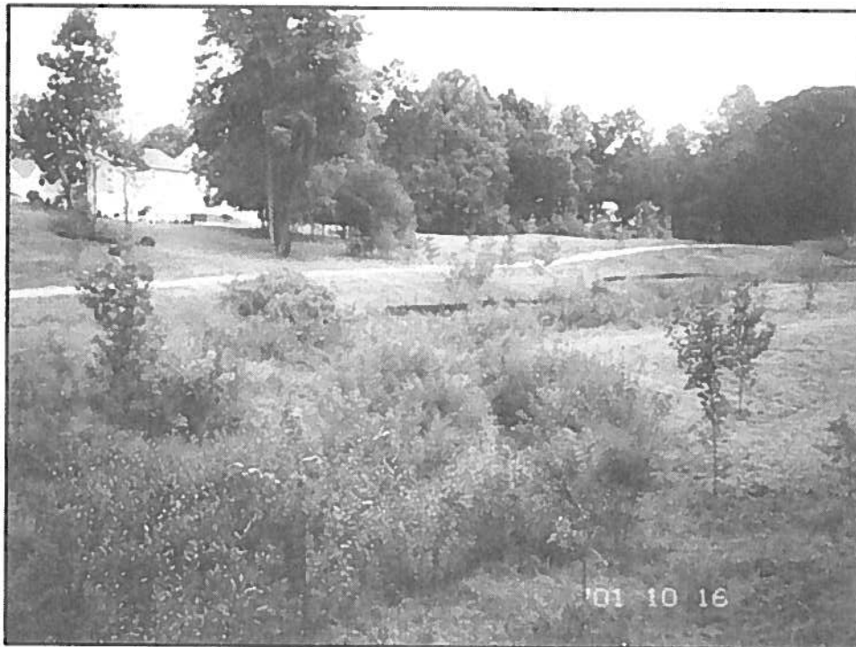
Photograph 2. Soil fabric lifts 17 months after construction.
