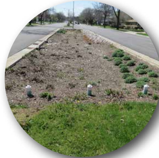
View of bioswales in median of Grange Avenue
