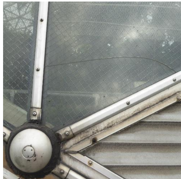
Figure 21. Cracked glass
