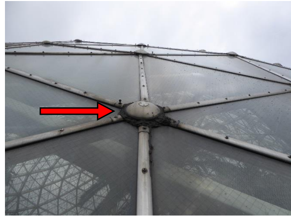
Figure 23. Sealant installed around hub of glass cladding
