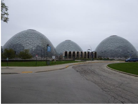
Figure 1. Overall view of the domes
