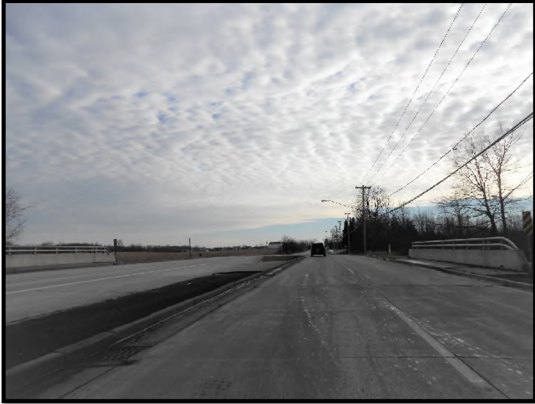
SOUTH VIEW OF 13 TH STREET, SUBJECT TO LEFT
