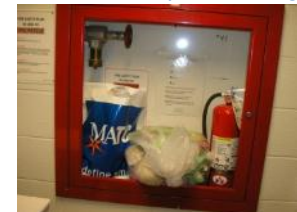
Fire extinguisher cabinet
