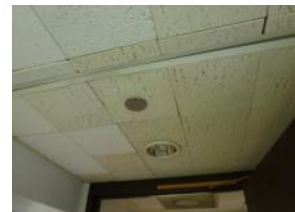
Recessed Downlight with Compact Fluorescent
