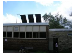
Unit vents outdoor air intake louvers
