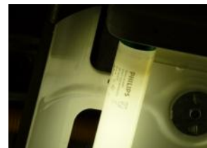
T-12 Fluorescent Lamp
