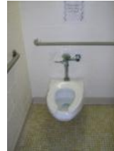
Wall mounted water closet
