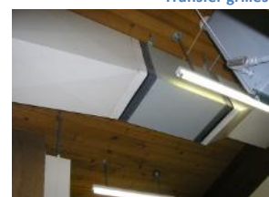
Transfer/exhaust in line fan
