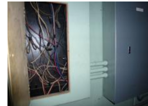
Panel Upgrade with Old Panel Converted to Splice Box
