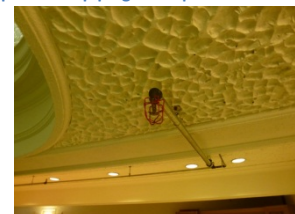
Downrigt sprinkler head with protection cover
