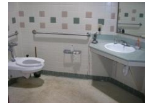
New plumbing fixtures are installed
