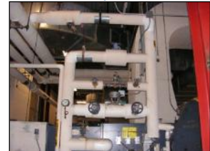
Pneumatic steam control valve
