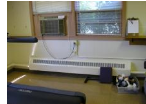
Window air conditioner/finned tube
