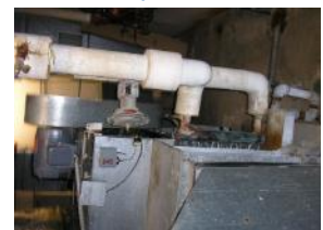
Control valve pneumatic actuator
