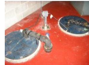
Trapped drain tile receiver (original to building)
