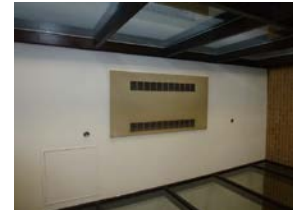
Ceiling cabinet unit heater
