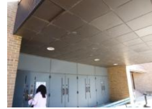
Recessed Light Fixtures
