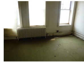
Cast iron radiator (2nd floor)
