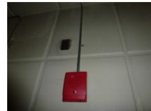
Fire Alarm Audio Device
