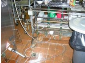
Original sanitary, vent, cold water piping (interior view)
