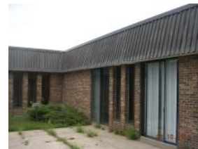
Landscape maintenance needed in interior courtyards
