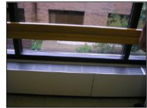
Perimeter finned tube radiation
