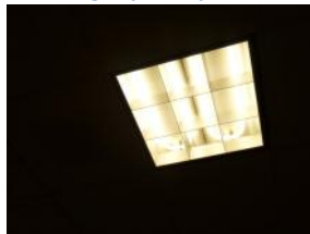
Parabolic Recessed Fluorescent Light Fixture
