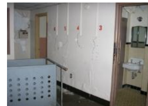
Lavatory in abandoned area
