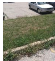
Overgrown grass, weeds in parking lot, landscaping on site needs grooming
