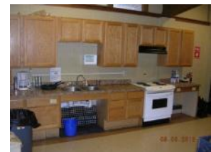
New kitchen casework with accessible counters, sink
