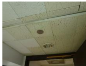
Concealed type sprinkler head
