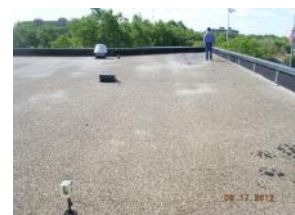
Roof generally in good condition
