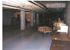
Lots of excess space is available in the basement for storage
