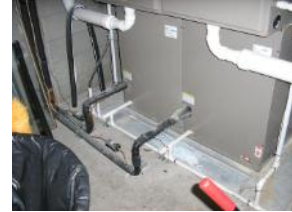
Lennox gas furnace unit (downflow)
