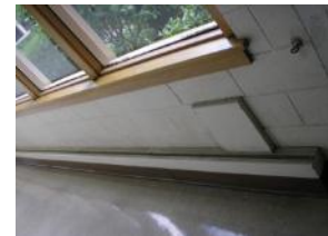
Finned tube radiation
