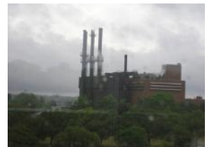
District heating/cooling plant
