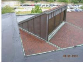
Asphalt shingles approx. 25 years old, generally in good condition
