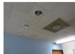
Room 1071 Existing Recessed Downlighting
