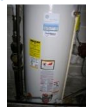
Gas fired heater is estimated to be 5+ and doesn't require replacement in the short term
