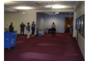
Administrative office area under renovation
