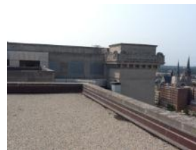
Roofs generally in good condition, some caulking needed at parapets
