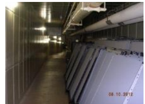
Basement contains good amount of storage space, cubicle partitions currently stored in corridor
