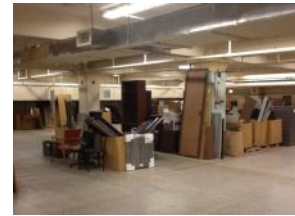
Basement storage area. A large amount of office furniture, workspace partitions, etc. are stored here
