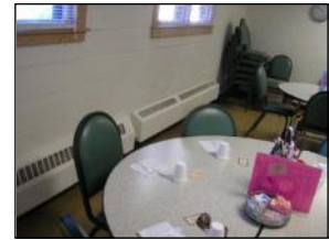
Finned tube radiation
