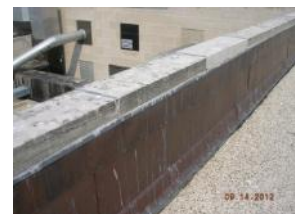
Parapets in good condition, some caulking needed
