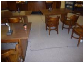
Microphone Wiring in Courtroom
