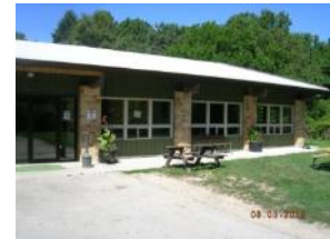
New roof recently installed
