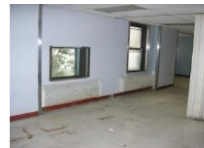
Finned tube radiation
