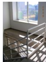
Typical stairwell, carpeted risers and landings in good condition
