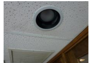
Incandescent Recessed Light Fixture
