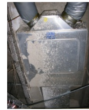
Dual duct mixing box
