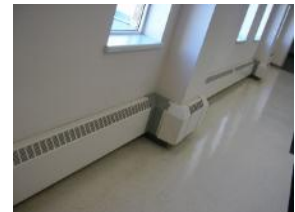
Finned tube radiation
