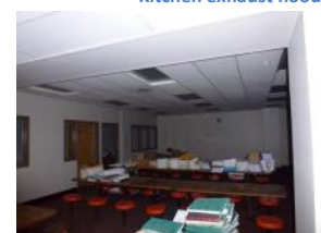
Existing Recessed Fluorescent Lighting
