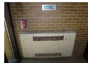
Wall cabinet unit heater
