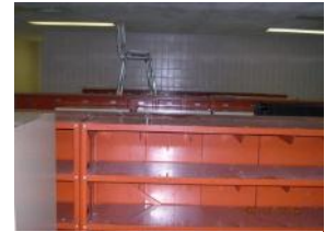
Locker room in good condition, currently utilized as storage space
