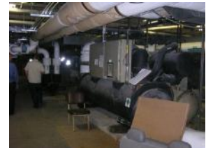
Centrifugal water chiller
