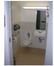
Typical public restroom on office floors
