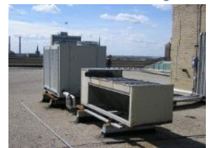
Air cooled condensing units
