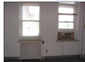
Operable window, steam radiator, and window air conditioner
