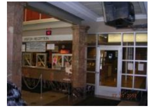
Floors, walls in public areas in good condition
