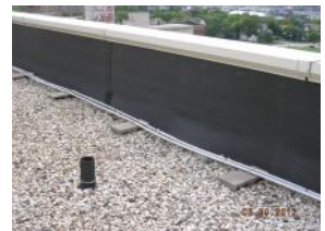
Roof generally in good condition
