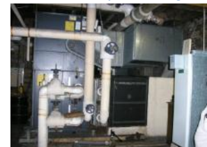
Modular air handling unit
