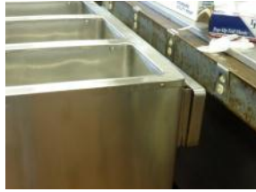
Receptacles (not GFCI)
