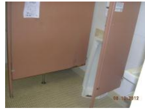
Typical restroom, in fair condition. Not fully HC accessible
