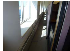
Finned tube radiation
