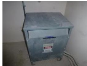
Step Down Transformer
