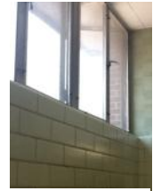
Operable windows, typical. Most are single pane glass windows
