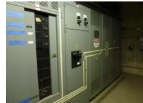
13kV Substation
