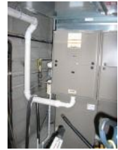
Lennox gas furnace unit (downflow)
