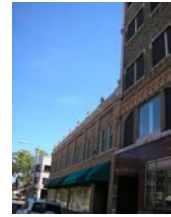
Existing Exterior of 2-Story Store Front
