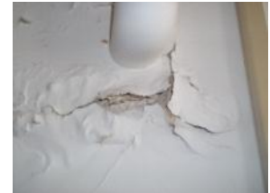
Water damage
