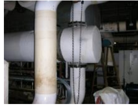
Shell and tube heat exchanger
