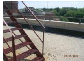
Roof and flashing generally in good condition
