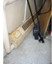
Finned tube radiation (janitors closet)
