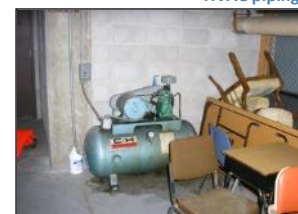
Temperature control air compressor
