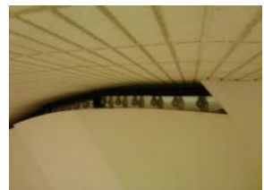
Incandescent Lighting in Auditorium
