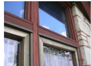
Wood frame windows, single pane
