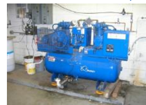
Temperature control air compressor
