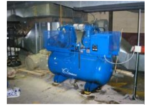
Temperature control air compressor
