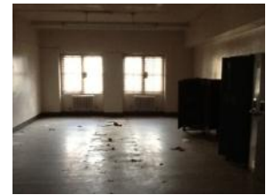
Typical room within the former jail block
