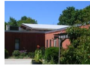
New roof recently installed above main hall
