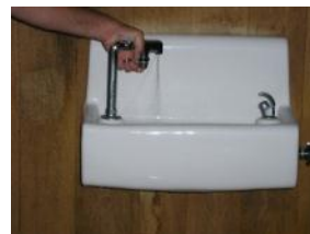
Drinking fountain (original to building)
