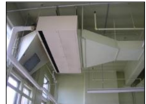
Steam horizontal unit ventilator
