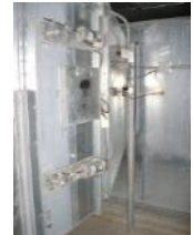
Control damper pneumatic actuators
