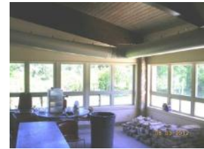
New 3-season room under construction
