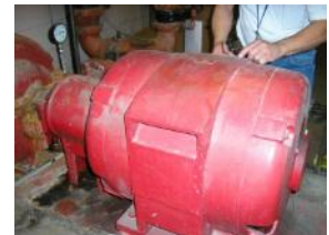
Routine in-house maintenance
