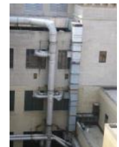
Light court exterior ductwork
