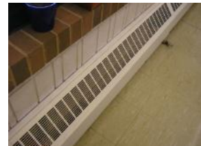
Finned tube radiation
