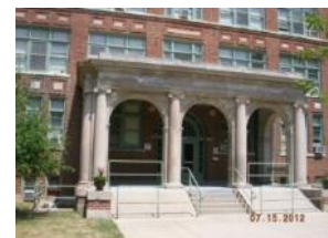
The main public entrance has great architectural character but is not handicapped accessible
