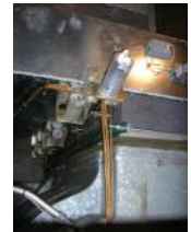
Control damper pneumatic actuators
