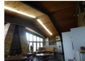
Existing Dining Hall Lighting
