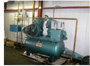
Temperature control air compressor
