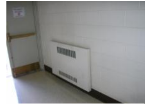
Wall cabinet unit heater
