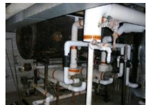
Abounded storage tank
