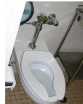
Wall mounted water closet
