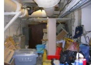
Basement corridors used as storage
