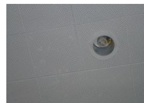
Recessed Downlight with Compact Fluorescent Lamp
