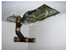
Exposed sanitary piping in the bathroom
