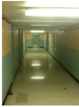
Typical corridor in basement
