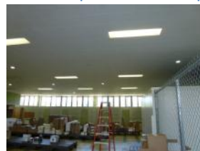
Existing Second Floor Lighting
