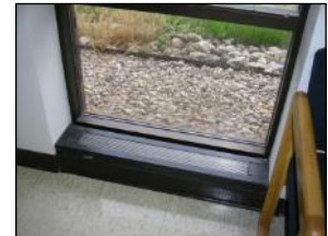
Sill mounted air cabinet (air baseboard)
