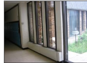
Perimeter finned tube radiation
