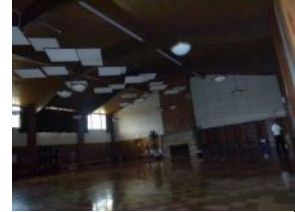
Main Hall Lighting
