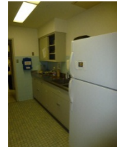
Two-compartment sink in pantry
