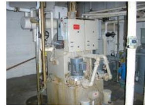
Vacuum condensate return pump
