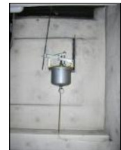
Pneumatic control damper actuator
