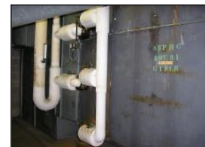
Chilled water cooling coil
