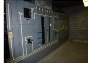
13kV Substation
