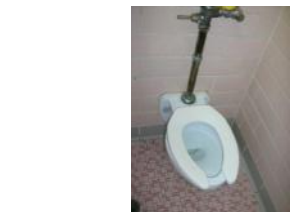
Wall mounted water closet
