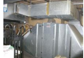
Air purification unit
