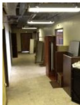
Corridor in the vacant 6th floor. Office furniture, equipment, etc. stored throughout the floor
