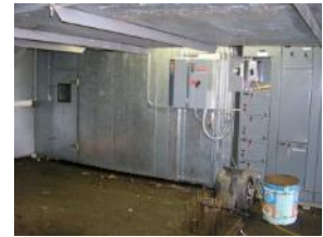
Modular air handling unit with variable frequency drive
