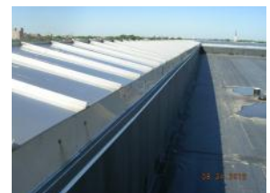
Roof recently replaced, in good condition
