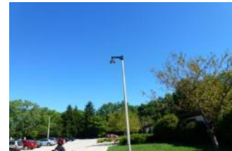
Parking Lot Light Pole
