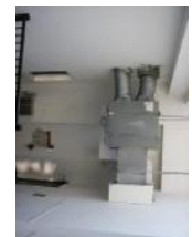
Dual duct mixing box
