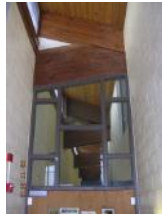
Exposed roof structure appears to be in good condition
