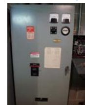
Generator Disconnect
