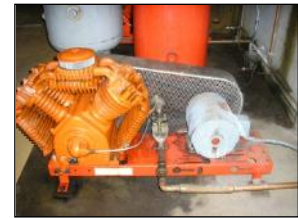
Temperature control air compressor
