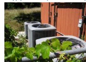
Lennox air cooled condensing units
