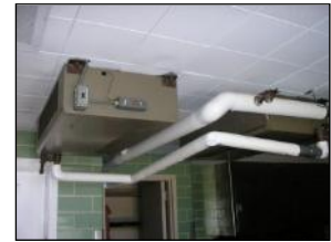
Ceiling cabinet unit heater
