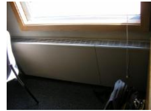
Finned tube radiation
