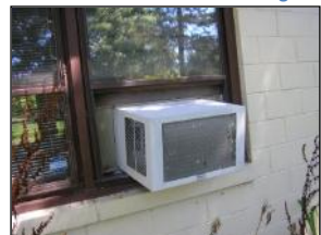
Window air conditioner
