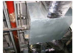
Dual duct mixing box
