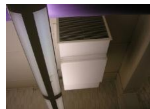
Return/relief/exhaust opening
