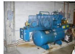
Temperature control air compressor
