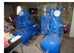
Temperature control air compressor
