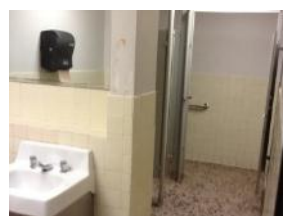
Public restrooms not fully HC accessible, are in fair condition
