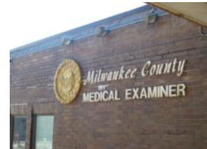
Exterior Light Fixtures
