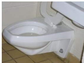
Wall mounted water closet
