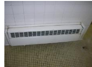
Finned tube radiation
