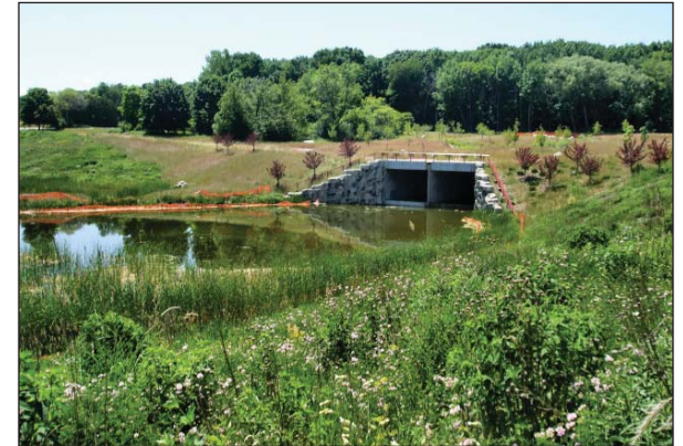
The MMSD Flood Management Basins serve the primary role of flood risk mitigation, while also creating vistas of the area's abundant natural features. Source: MMSD
