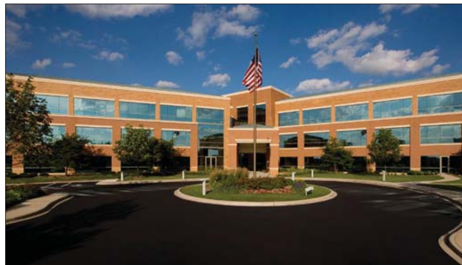
A 203,000-square-foot office building fronts the western side of I-41/US45 at the MCRP. While the four stories rise above the highway and begin to frame a skyline, the potential exists to add density and height. Opportunities for infill development could satisfy the desires of this Plan and the MCRP’s original master plan to add mixed uses and public places. Source: Irgens
