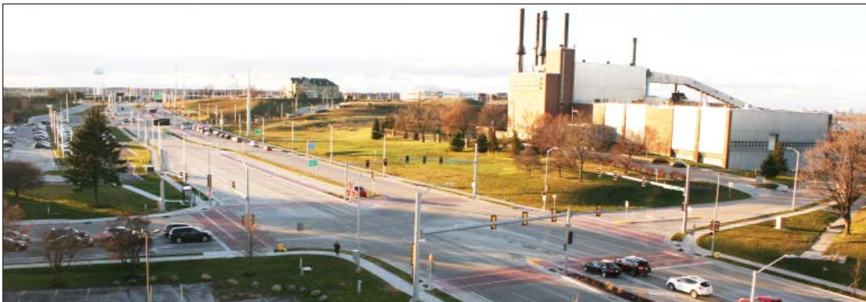
Watertown Plank Road looking west at 92nd Street. Source: GRAEF
