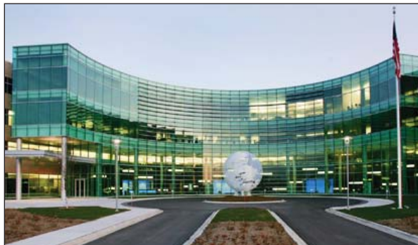
GE Healthcare is a major employer at the Milwaukee County Research Park. The company's building is a showcase of its innovative technologies and services. Source: Irgens
