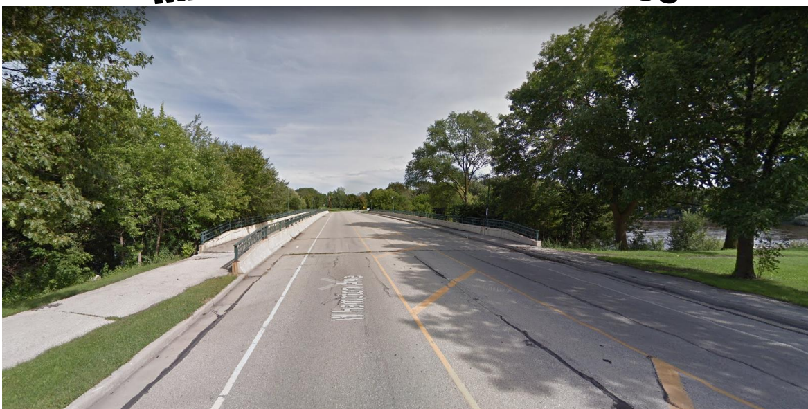
<Image Capture of Existing Condition within Lincoln Park Looking East-Sept 2018 @ 2019 Google>
