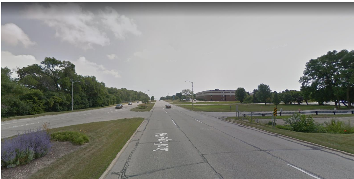
<Image Capture of Existing Condition 1600 feet east of Teutonia Ave. Looking East-Nov 2016 @ 2019 Google>
