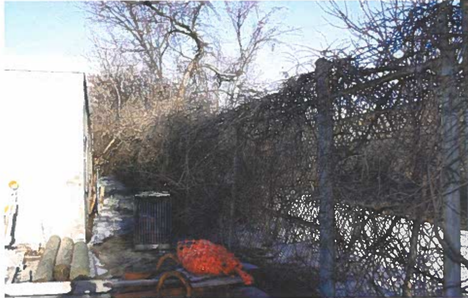
South yard freeway edge condition.
