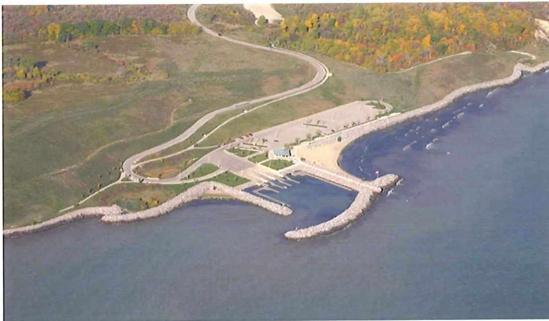
Figure 1. Aerial View of Bender Park
