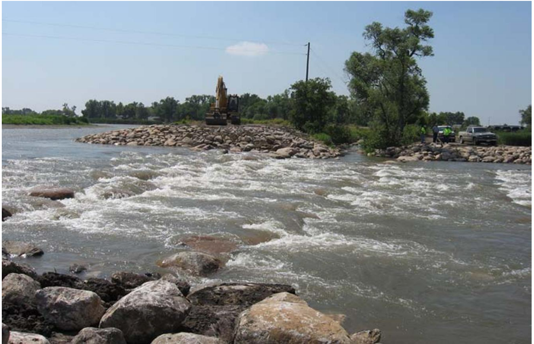
Figure 91. Rapids replacing dam to provide grade control and facilitate fish and canoe passage. Reconnecting Rivers: Natural Channel Design in Dam Removals and Fish Passage , p. 80. Minnesota Department of Natural Resources Ecological Resources Division, 2010.
