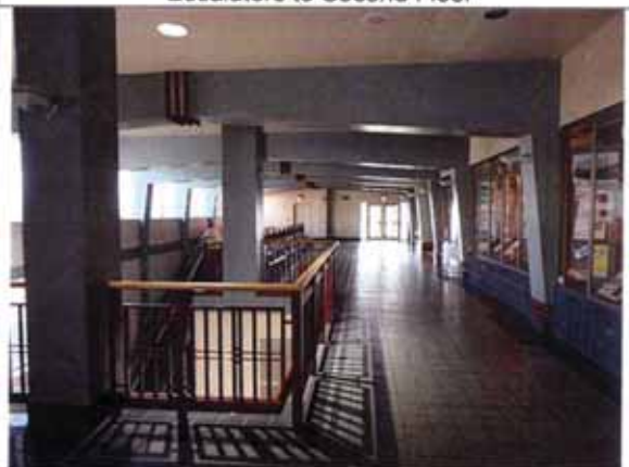
Second Floor Common Area
