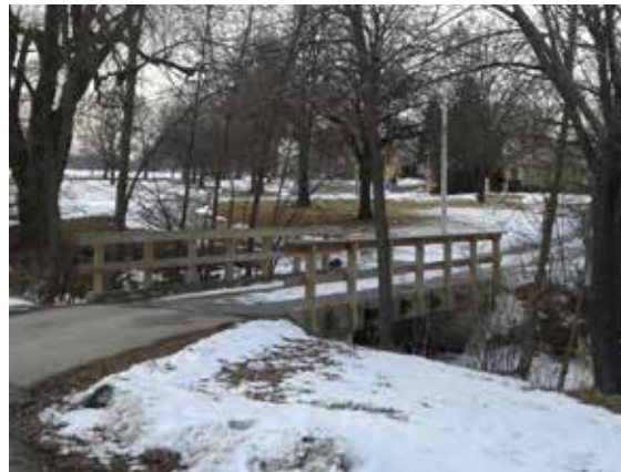
View of existing pedestrian bridge crossing looking northeast
