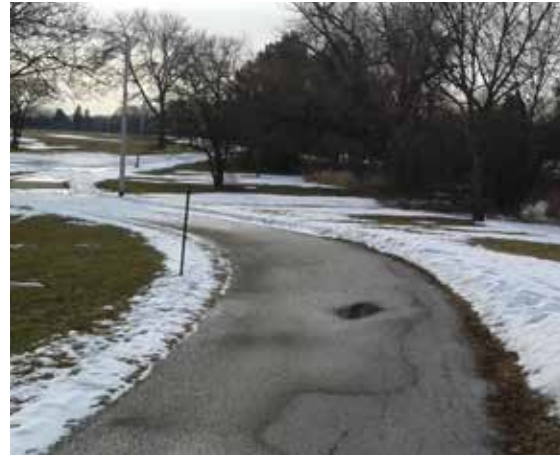
View of existing asphalt pathway looking northeast
