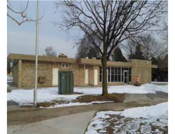
View of existing park bathhouse looking east
