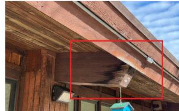
DETERIORATED ROOFING & EAVES
