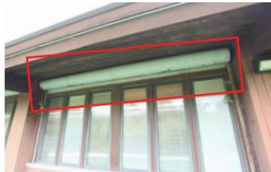
MALFUNCTIONING SECURITY LOUVERS
