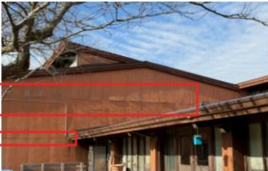
DETERIORATED SIDING - MULTIPLE LOCATIONS
