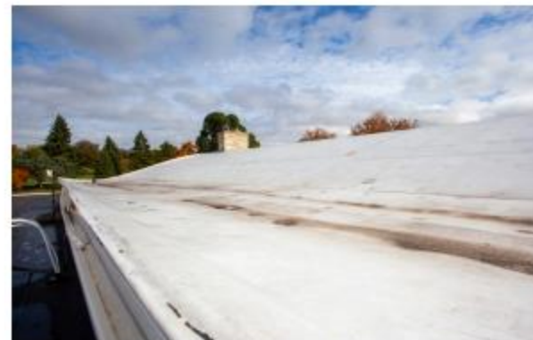
ROOFING MEMBRANE AT END OF USEFUL LIFE & FREQUENTLY LEAKS
