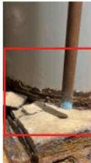
RUSTING MECHANICAL SYSTEMS-EVIDENCE OF REPEATED FLOODING IN BASEMENT
