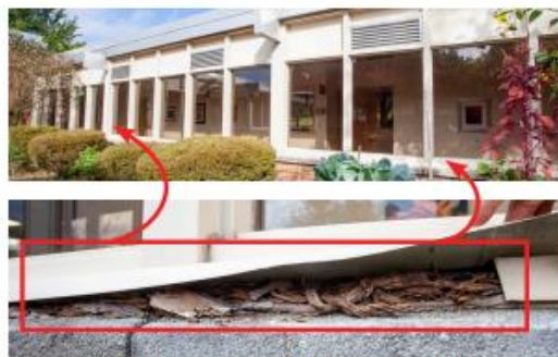
ROTTED WINDOWS-TYPICAL ON ALL WINDOWS AT WASHINGTON PARK
