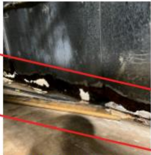
RUSTING MECHANICAL SYSTEMS-EVIDENCE OF REPEATED FLOODING IN BASEMENT
