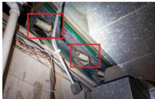
DISCONNECTED GEARS TO OPERATE/OPEN LOUVERS FOR HVAC
