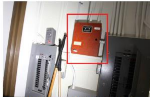
DEFECTIVE ALARM SYSTEM: TYPICAL OF MCGOVERN, WILSON, KELLY, & WASHINGTON PARK
