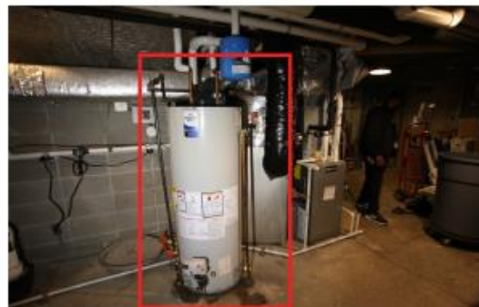
WATER HEATER - END OF USEFUL LIFE
