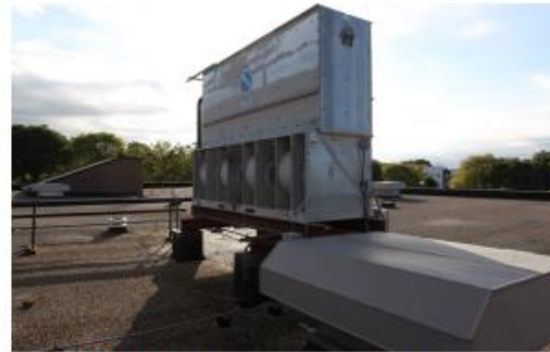
ROOFTOP COOLING TOWERS - NEARING END OF LIFE USE
