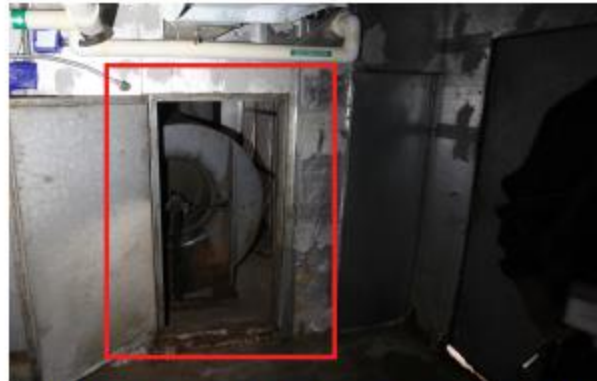
DAMAGED AIR EXCHANGING FAN DOESN'T WORK
