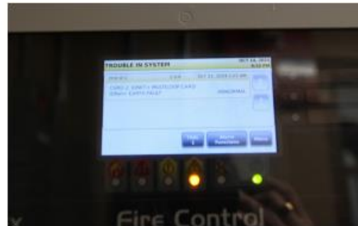
FIRE ALARM PANEL WITH TROUBLE CODE SHOWN
