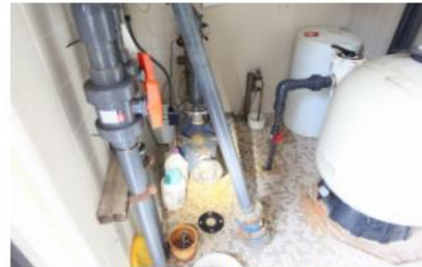
SPLASHPAD FILTRATION EQUIPMENT DETERIORATED & NEARING END OF LIFE CYCLE
