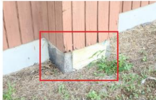
MISSING INSULATION AT FOUNDATION
