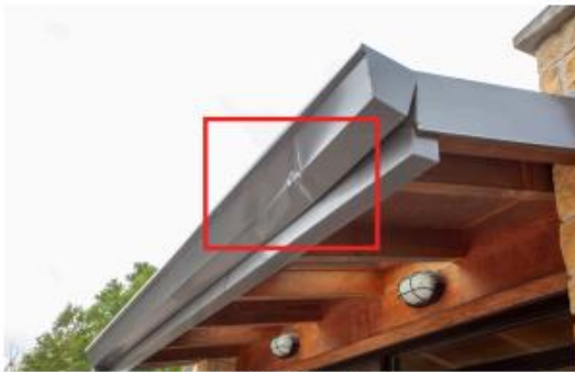
DAMAGED GUTTERS
