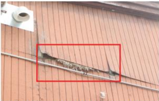
WILDLIFE NESTING IN DETERIORATED SIDING
