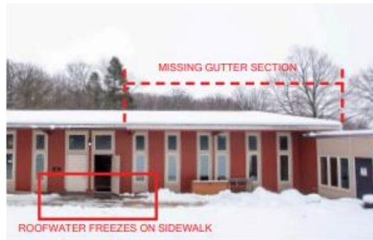
MISSING & INEFFECTIVE GUTTERS LEAD TO ICE DAMING, ROOF DAMAGE, & SLIPPERY WALKWAYS
