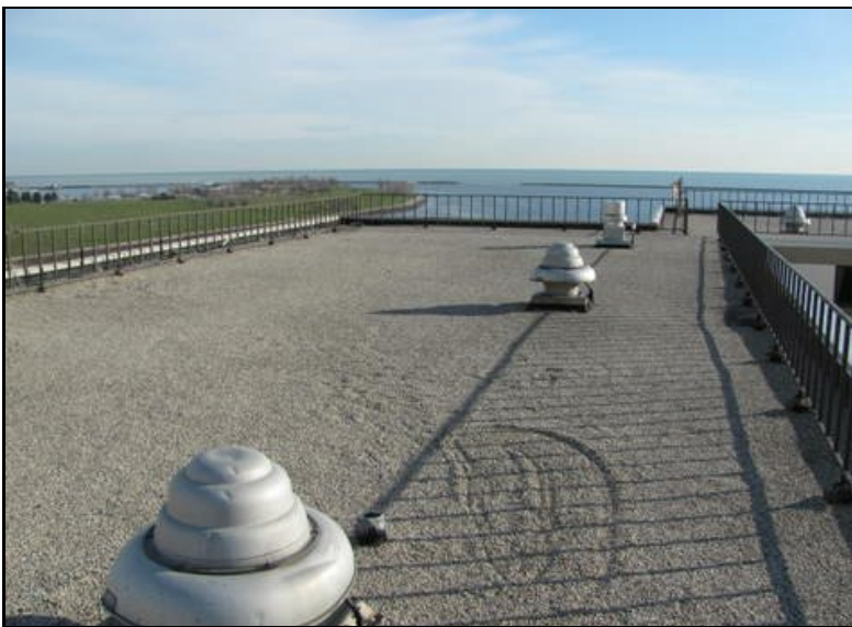
War Memorial built-up roof
