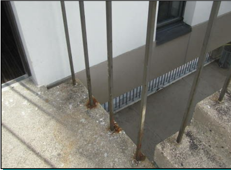
Railing deterioration
