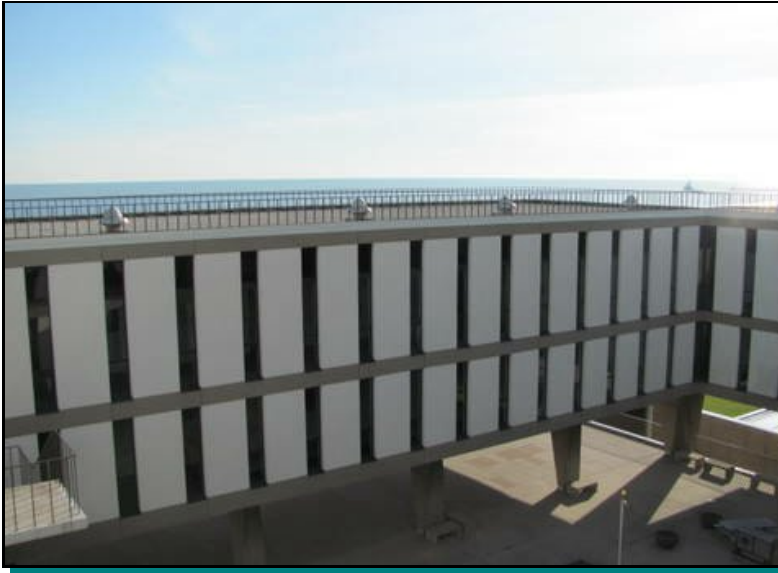
EIFS facade at War Memorial courtyard
