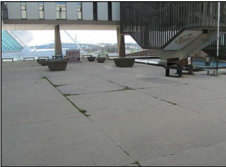
Concrete deterioration
