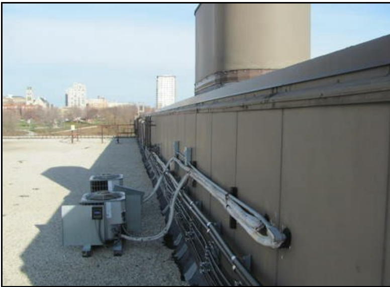
Metal siding at penthouse
