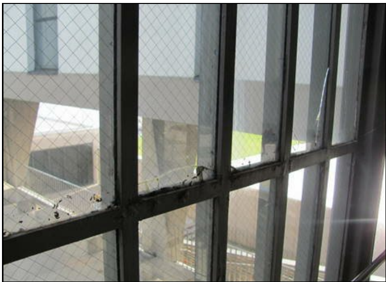
Frame deterioration
