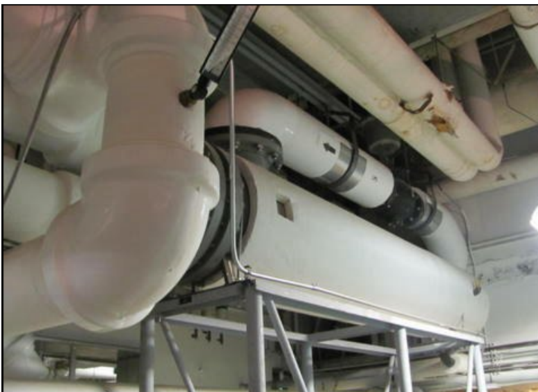
Building heat heat exchanger
