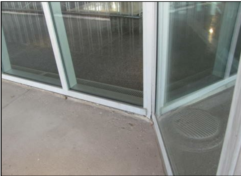
Frame deterioration
