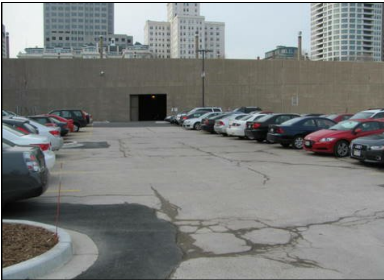
Pavement deterioration
