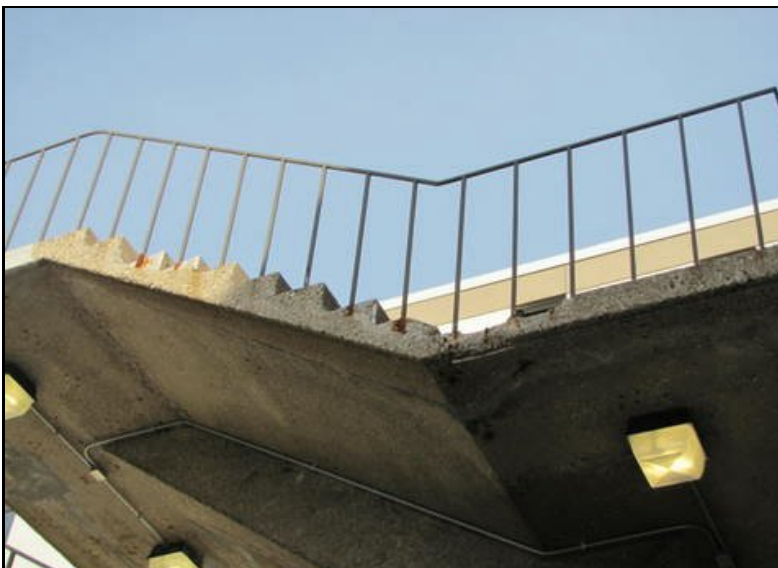
Concrete deterioration
