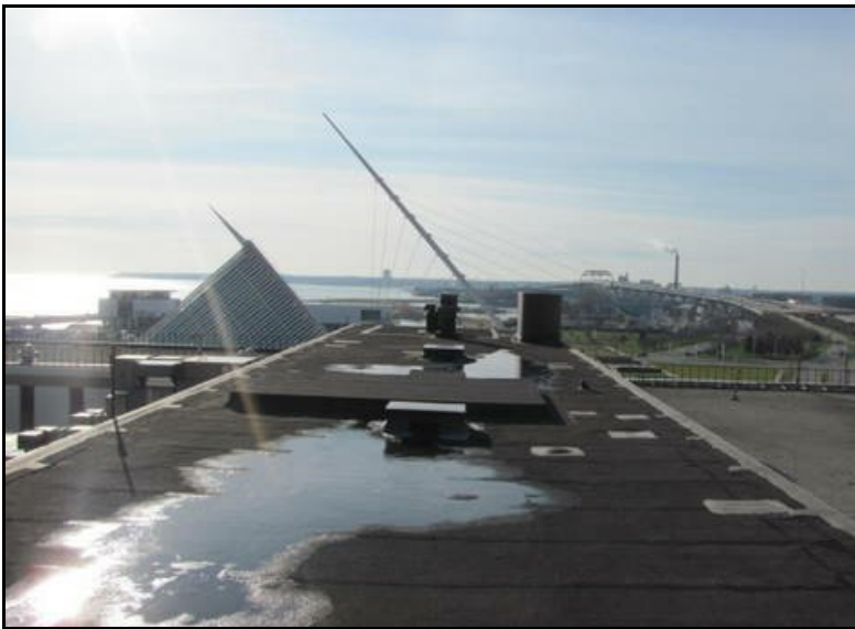
Penthouse modified bitumen roof
