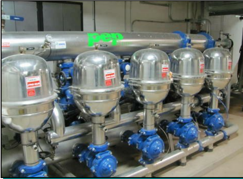
Lake water filtration equipment
