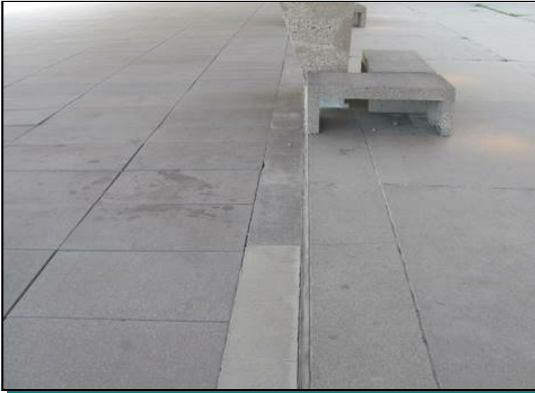
East expansion joint
