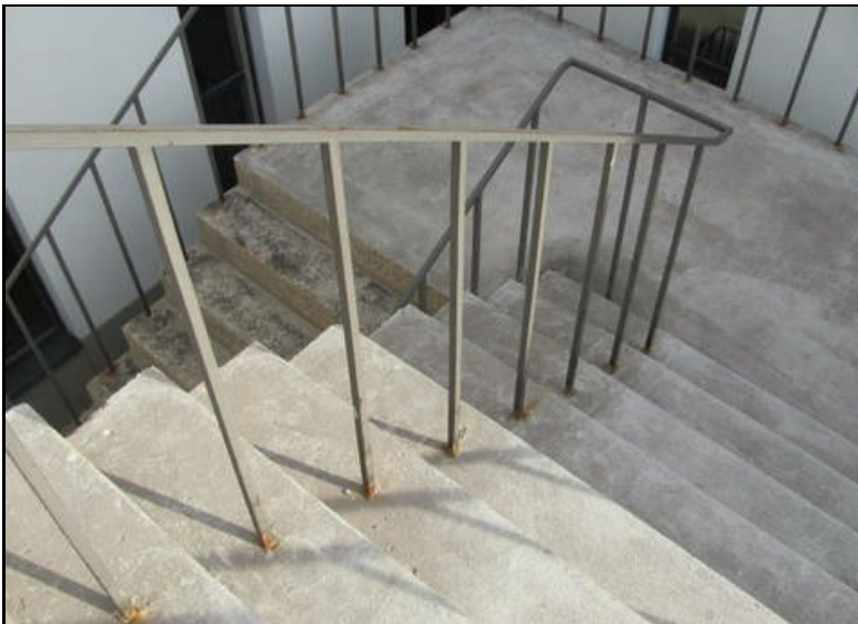
Railing deterioration
