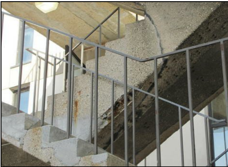
Concrete deterioration
