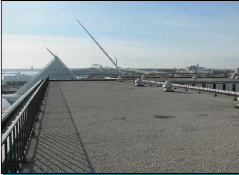
War Memorial built-up roof
