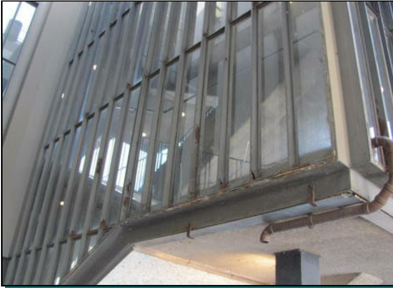
Frame deterioration
