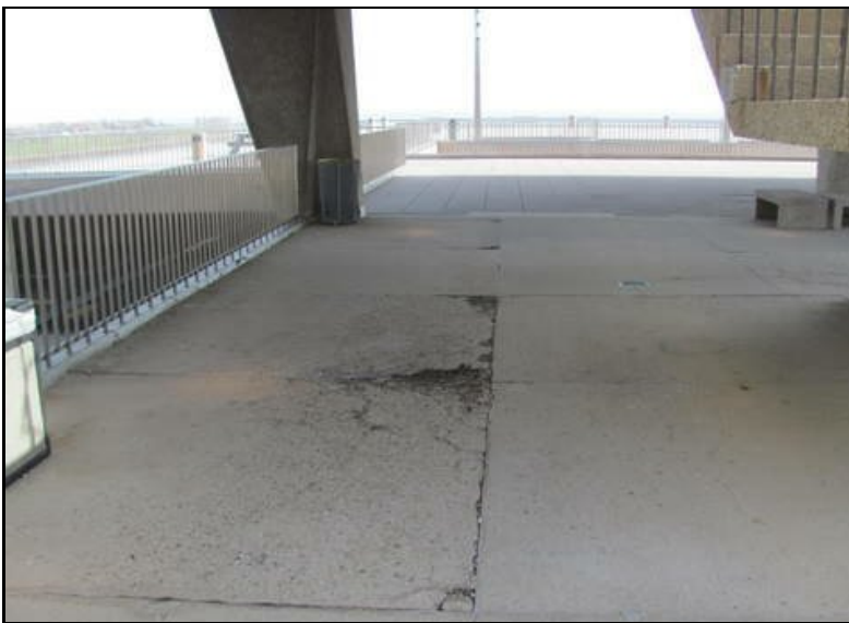
Concrete deterioration
