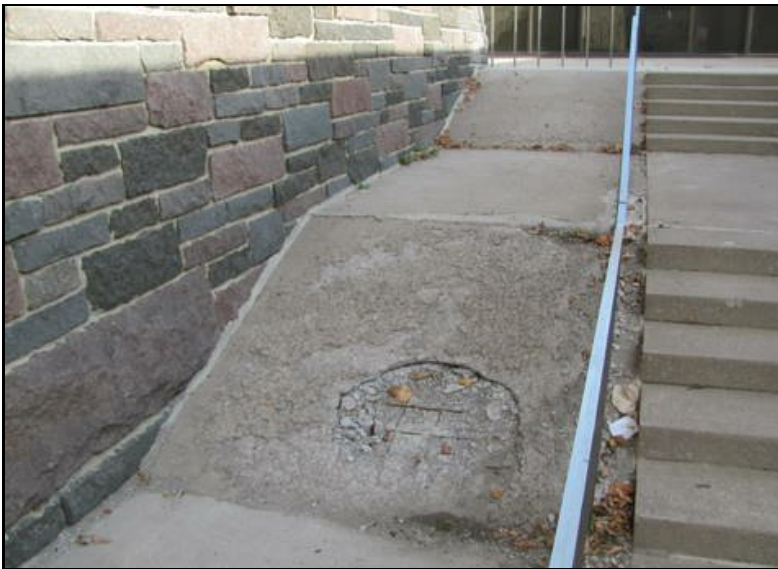
Concrete deterioration
