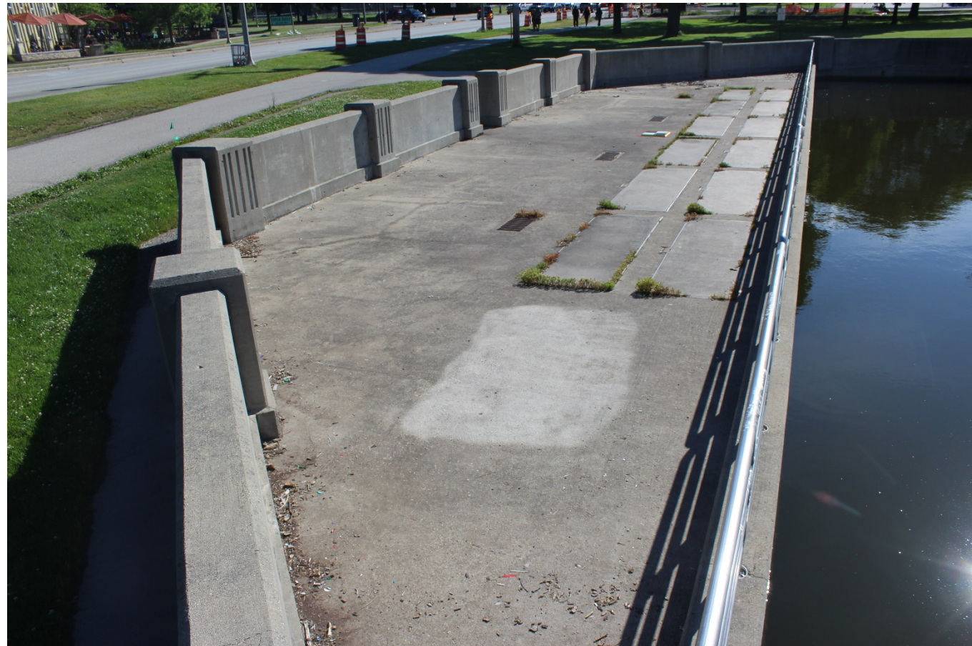
EXISTING HEADWALL AND PARAPET WALL
